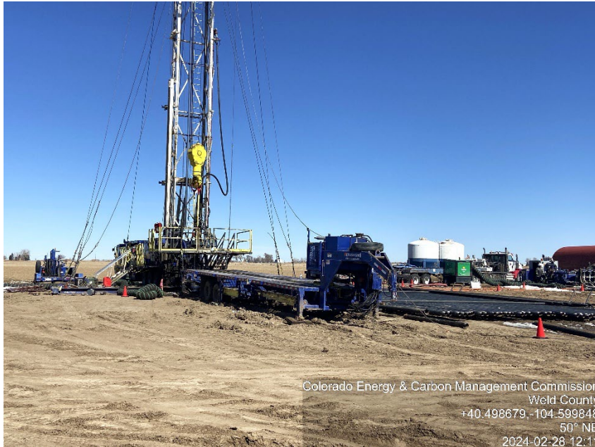
Photo #1 Ehrlich #1 (123-12382) Wellsite Plugged & Abandoned | PA Plugging Ops; Cementing: stub-plug
