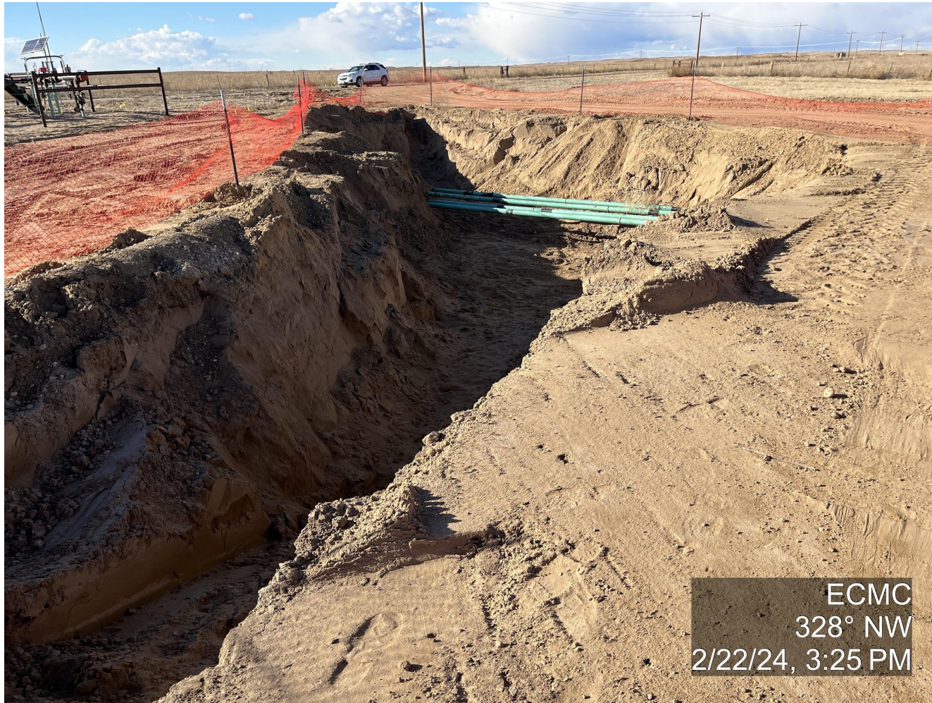
Photo 5. The photo was taken at the well location facing Northwest. The photo illustrates the active excavation of a reported spill on the facility production pad.
