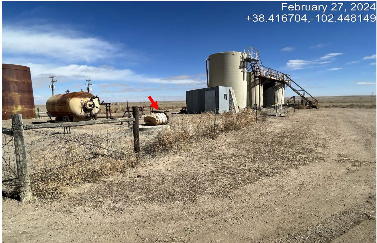
Photo 3. Facing northeast at the backside of the tank battery. The secondary containment at the red arrow has tipped over.
