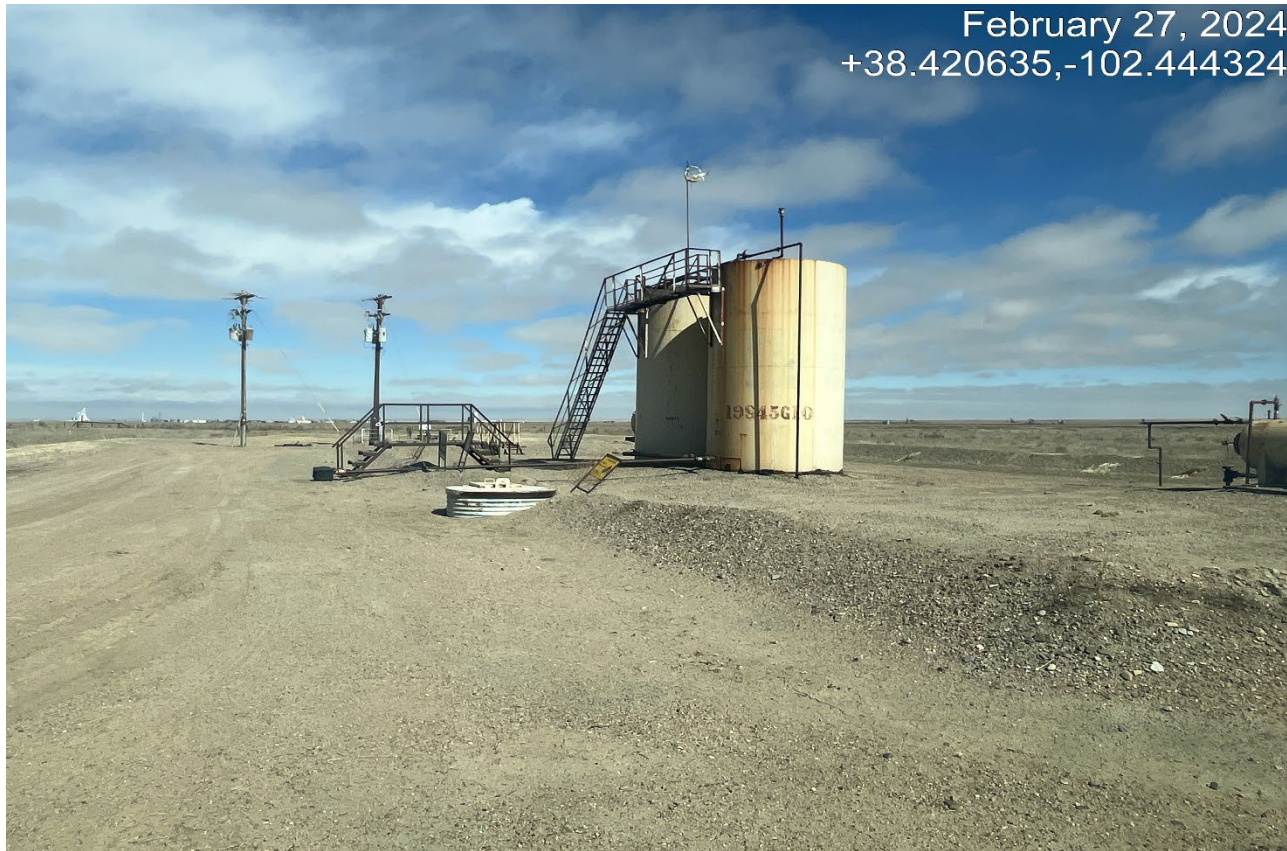
Photo 2. Facing northeast towards the tank battery. The wind sock for H2s needs to be replaced.
