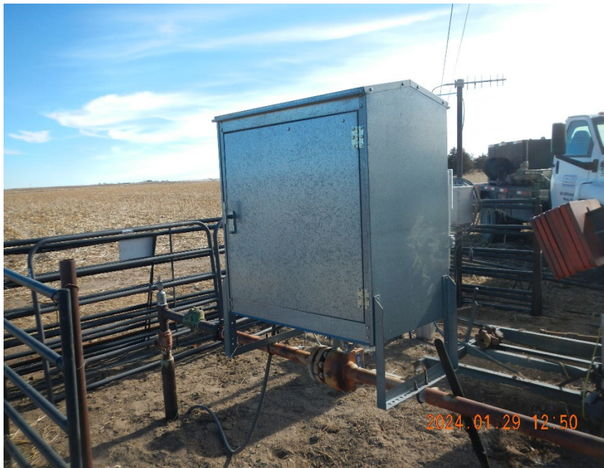
5. View of flowline mounted meter run box.
