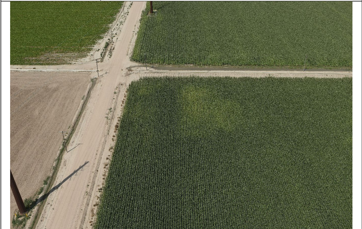
In View – Tank Battery, Access Road, Flowline NORTH – 40.445212 / -104.667934
