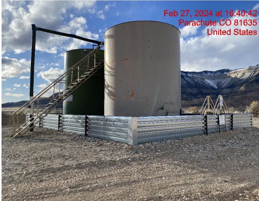
Tank Battery/Tank Missing Labeling – Photo #09623
