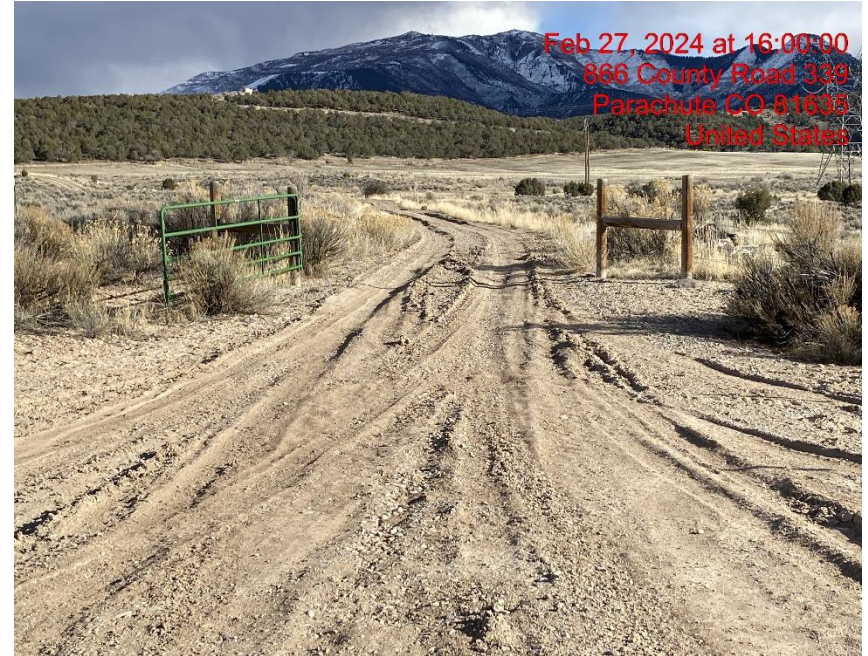
Insufficient Vehicle Tracking BMPs at Location Entrance/Exit – Photo #09612
