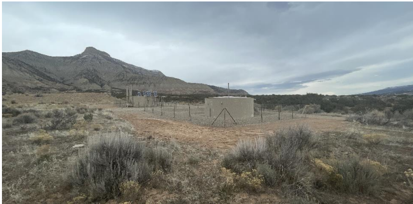
South West corner of location.
