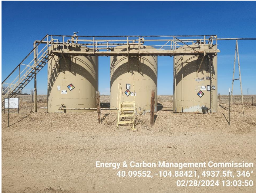
Photo 9 Tank Battery.
