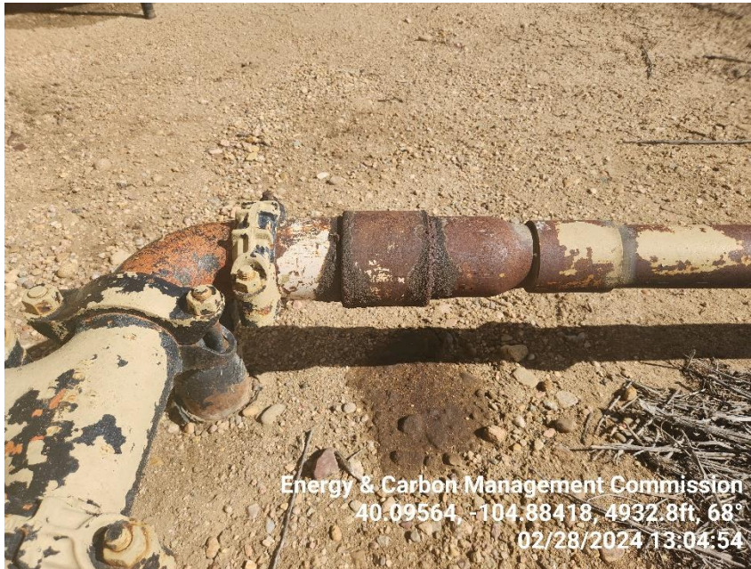
Photo 13 Stained soil under west crude tank flow line.
