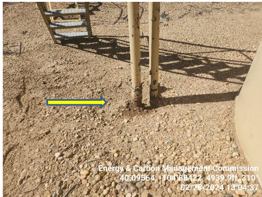
Photo 11 Stained soil around west crude tank flow line.
