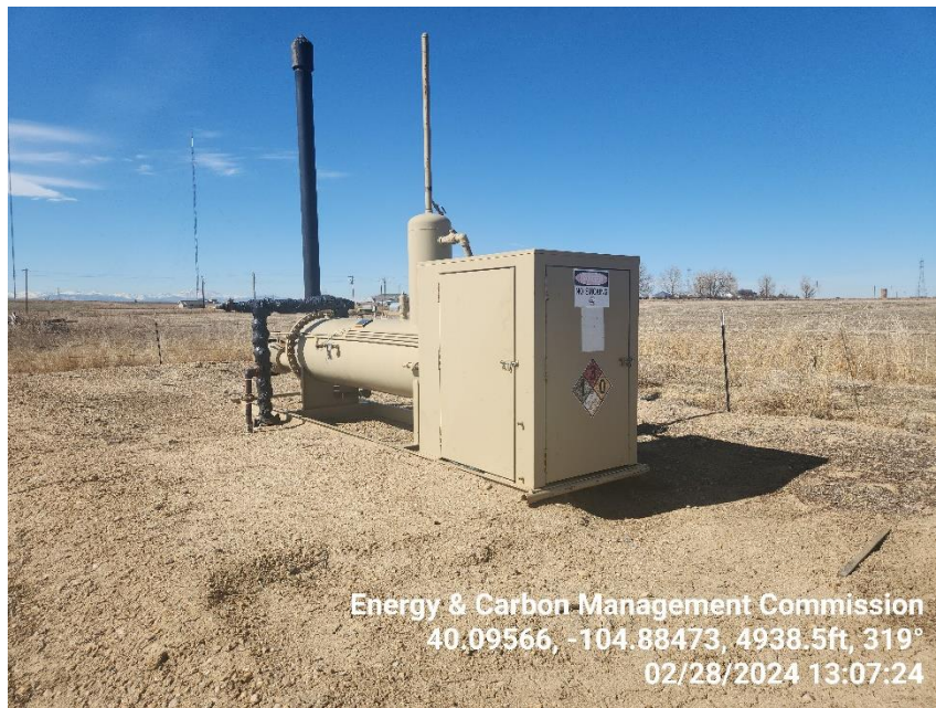
Photo 15 Horizontal Heated Separator.
