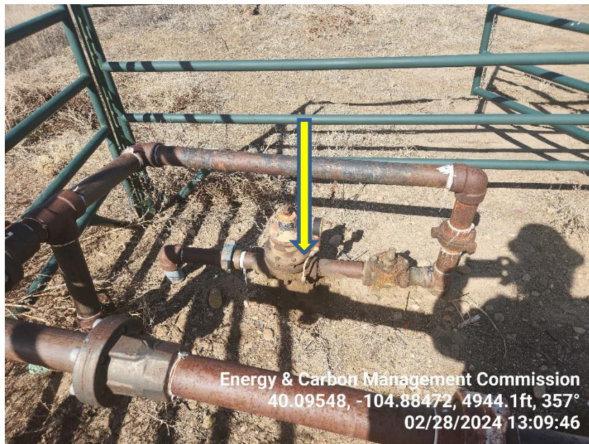
Photo 17 Stained soil by the Gas Meter Run flow line.
