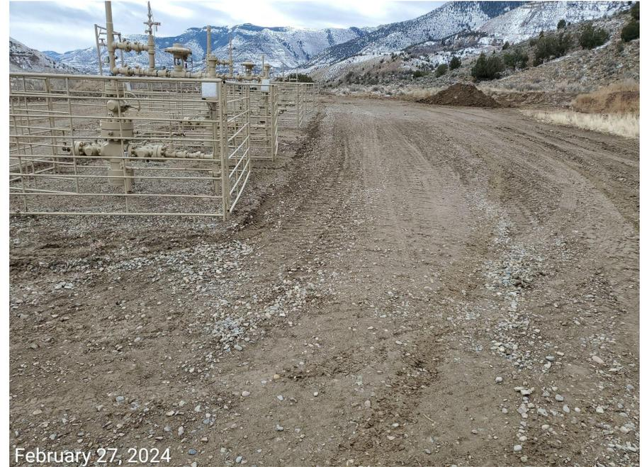
**Photo 4:** Photos taken from the working pad surface. BMPs to stabilize the working pad surface appears to have been maintained; additional compaction is apparent, and potentially addition of road base material. Continue to monitor and maintain BMPs to ensure location remains stabilized.
