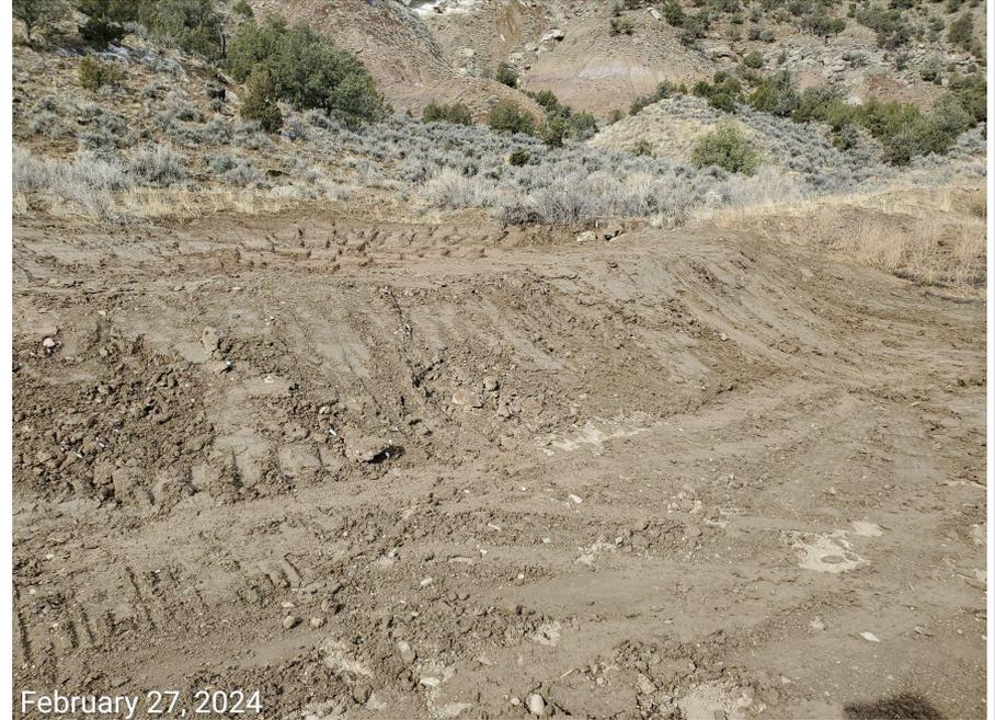
**Photo 2:** Photos taken from the sediment trap on the west end of the Location. Sediment material has been removed from the BMP and berms have been maintained.
