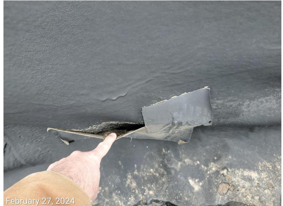
**Photo 6:** See comments under photo 5. Photo right example showing patches from previous repair work have not been maintained.
