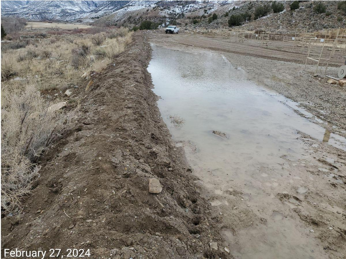
**Photo 9:** Photo taken from the east end of the working pad surface, facing south. Photo shows stormwater ponding has persisted on the east end of the Pad.
