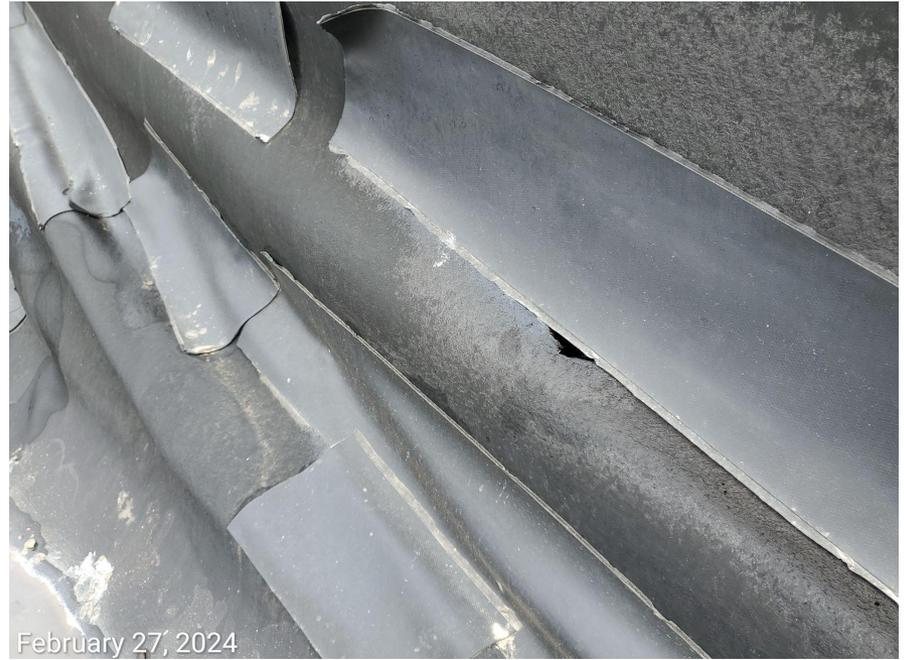
**Photo 5:** Photos 5-6 taken from the tank battery facility. Photos examples showing holes and tears remain apparent within the liner of the secondary containment measure.
