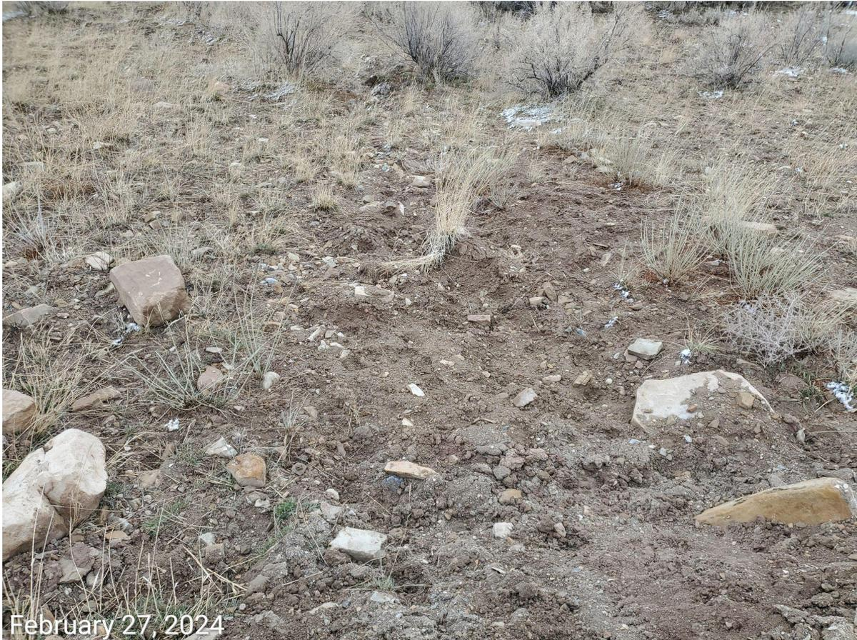
**Photo 8:** Photo taken from the slopes on the east end of the Location. Operator appears to have placed additional soil to repair the erosion degradation observed on the slopes on the east end of the Location. BMPs to stabilize the soils not observed per the CA. Unclear if additional reclamation work, such as seeding, has been performed.
