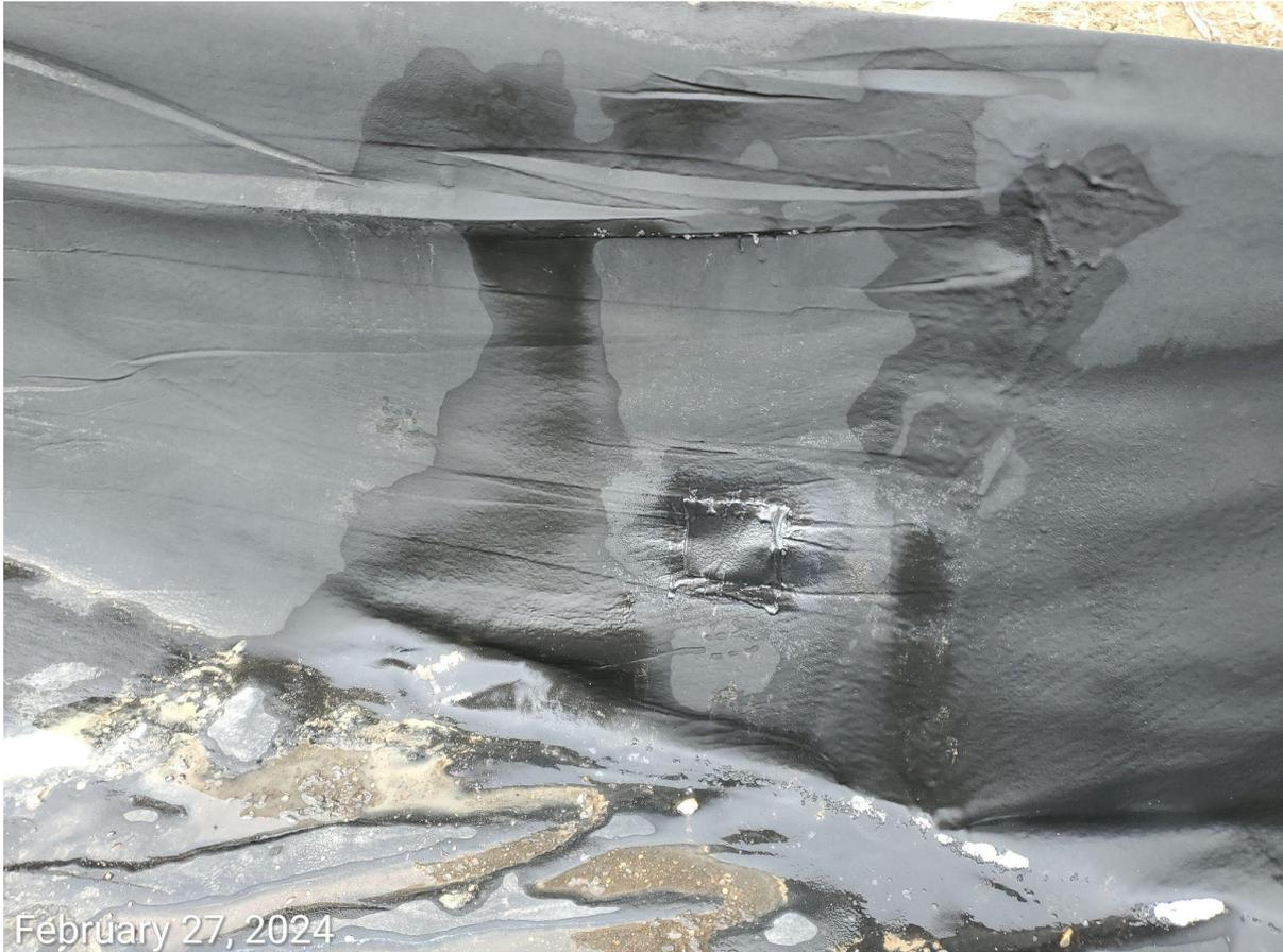
**Photo 7:** Photo example showing Operator appears to have conducted some maintenance work at the containment measure. Work is insufficient as holes/tears remain.
