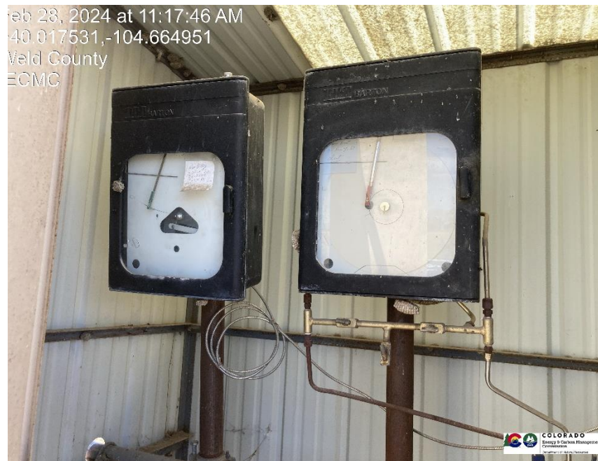
Pic 3 GMR has not been calibrated, no chart available.
