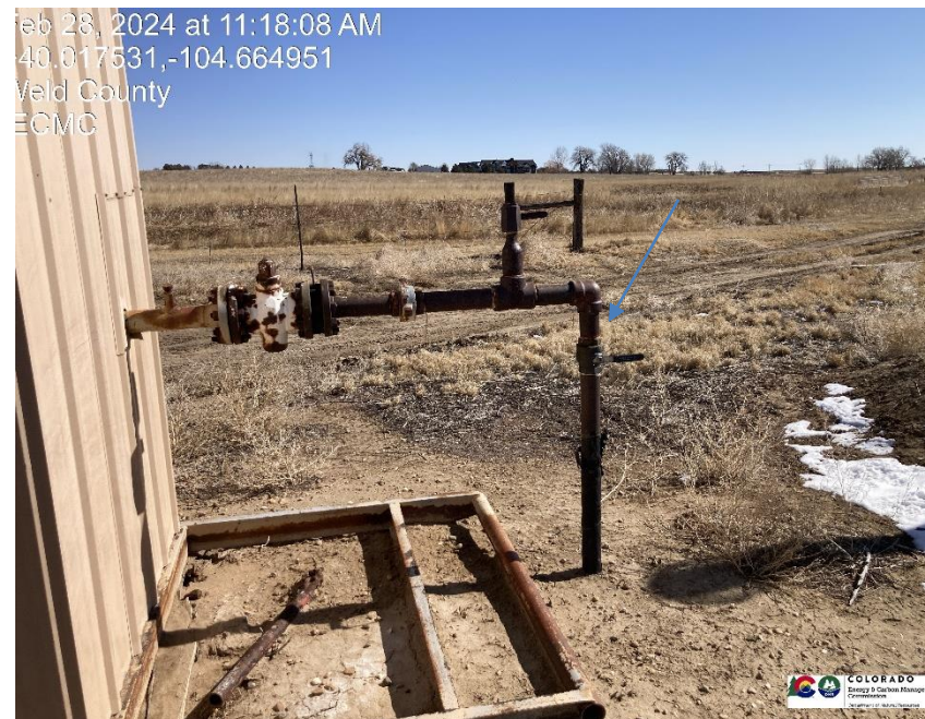
Pic 4 gas sales line appears to be in the close position.
