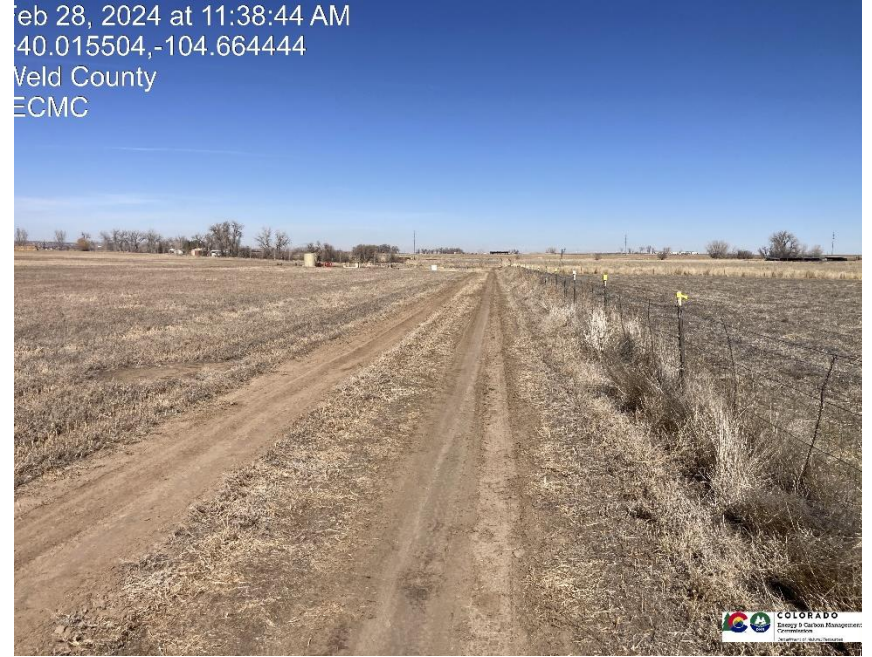
Pic 17 lease road control measures are not maintained, overgrown with vegetation.
