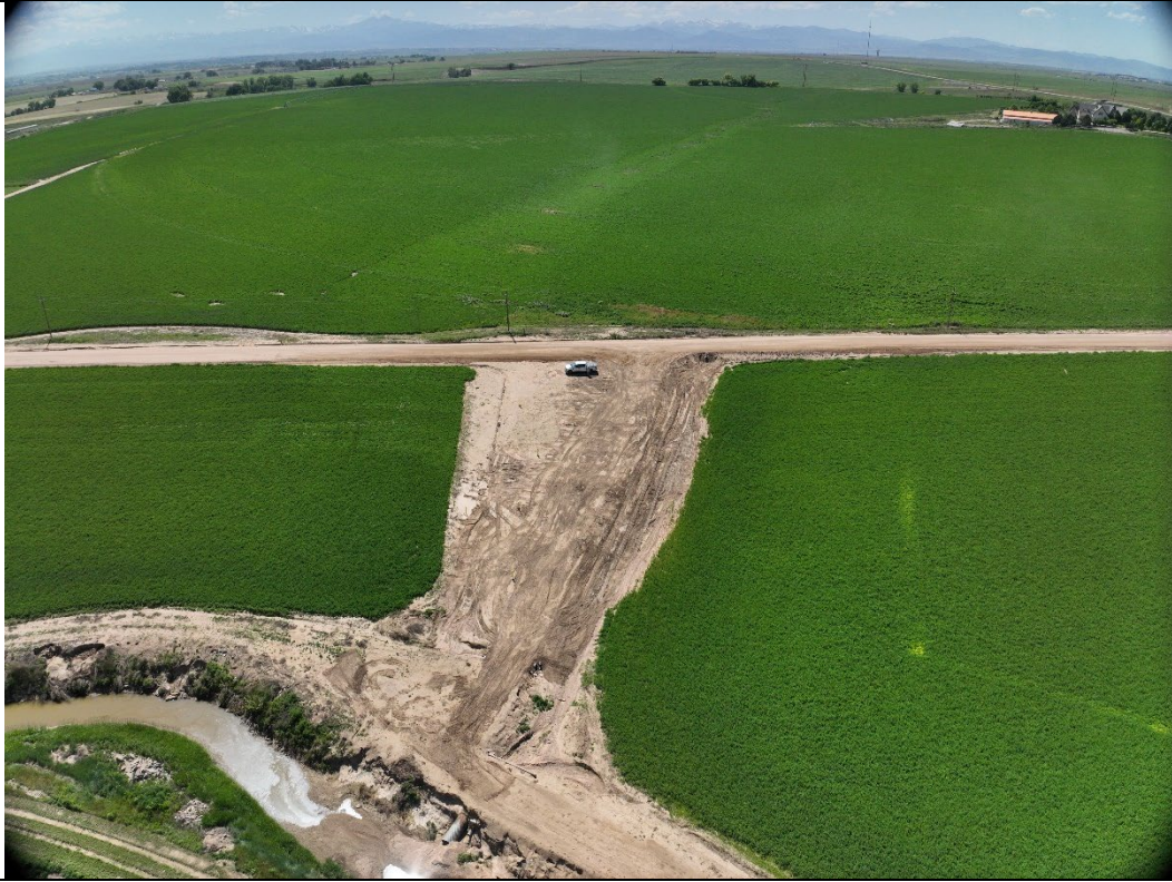
In View – Tank Battery, Flowline
