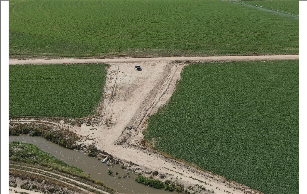
In View – Tank Battery, Flowline
