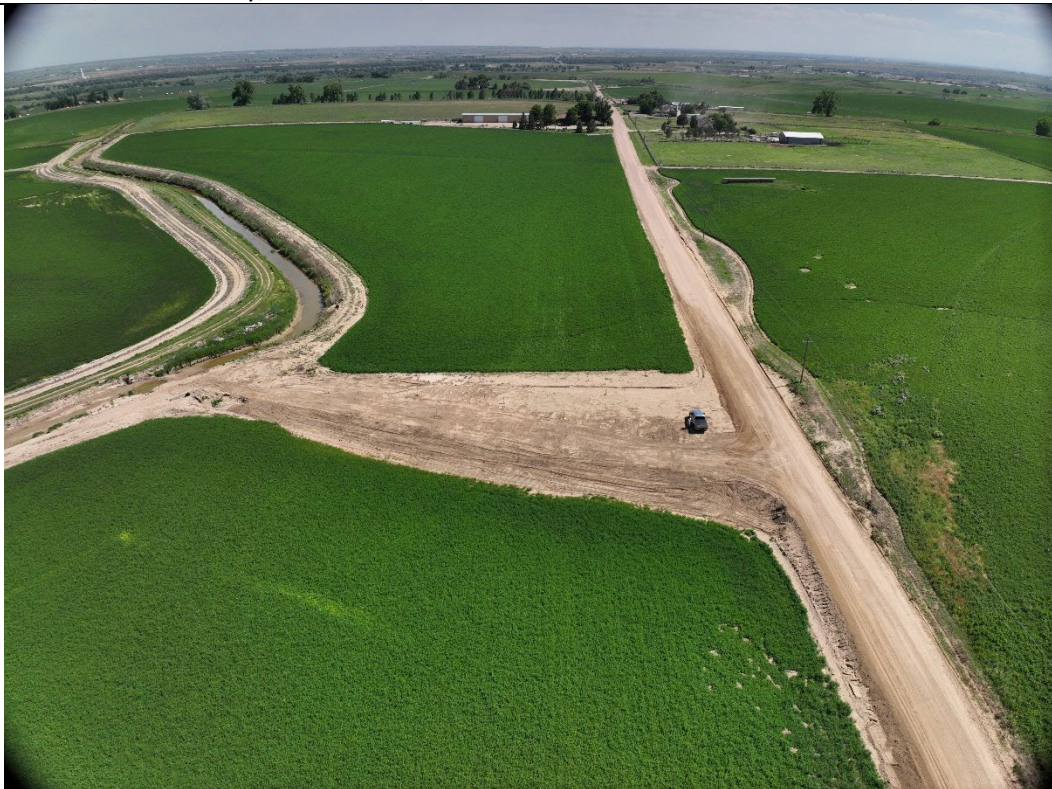
In View – Tank Battery, Flowline
