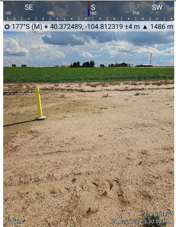
Looking South at tank battery and separator location – 40.372489 / -104.812319
