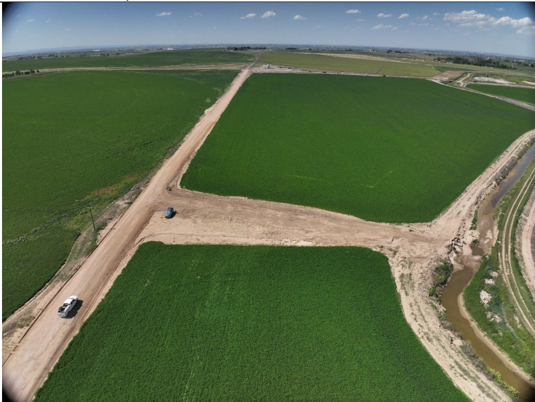
In View – Tank Battery, Flowline
