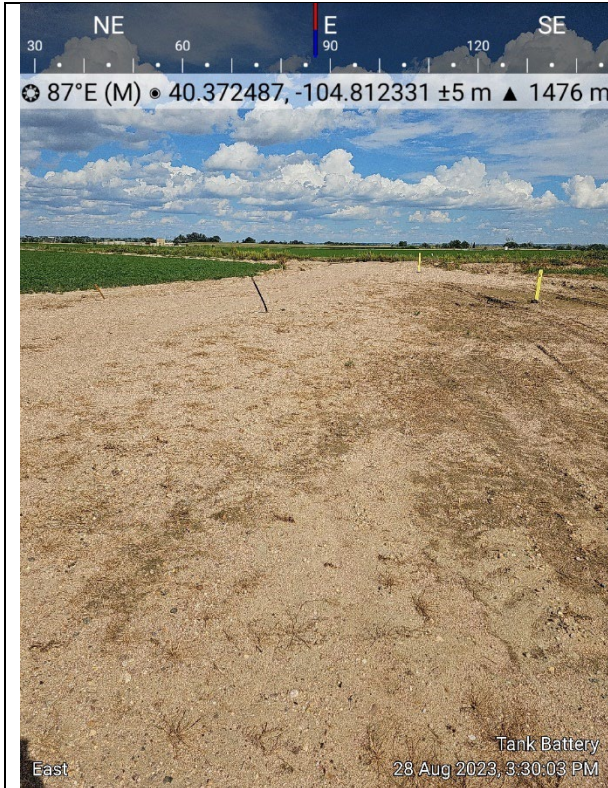
Looking East at tank battery and separator location – 40.372487 / -104.812331
