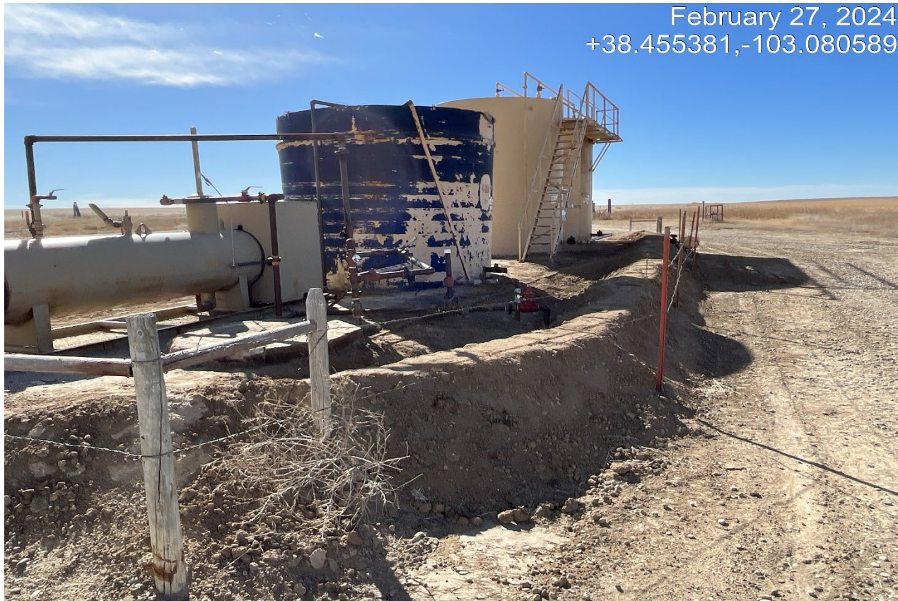
Photo 3. Facing south toward the tank battery. The secondary containment has been repaired.
