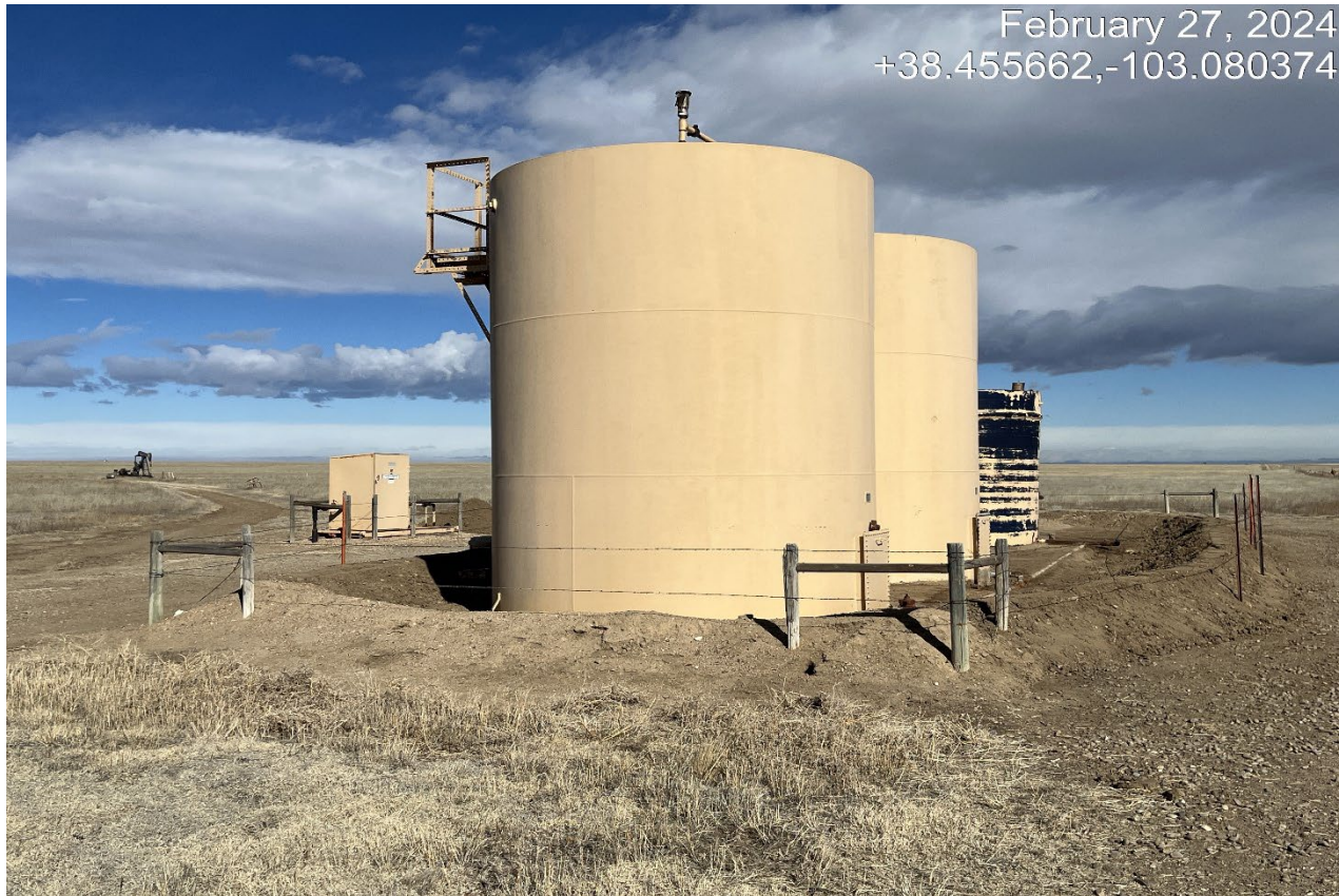
Photo 2. The fence around the tank has been repaired. The wires are tight however there are only 2 wires which may not keep livestock out.
