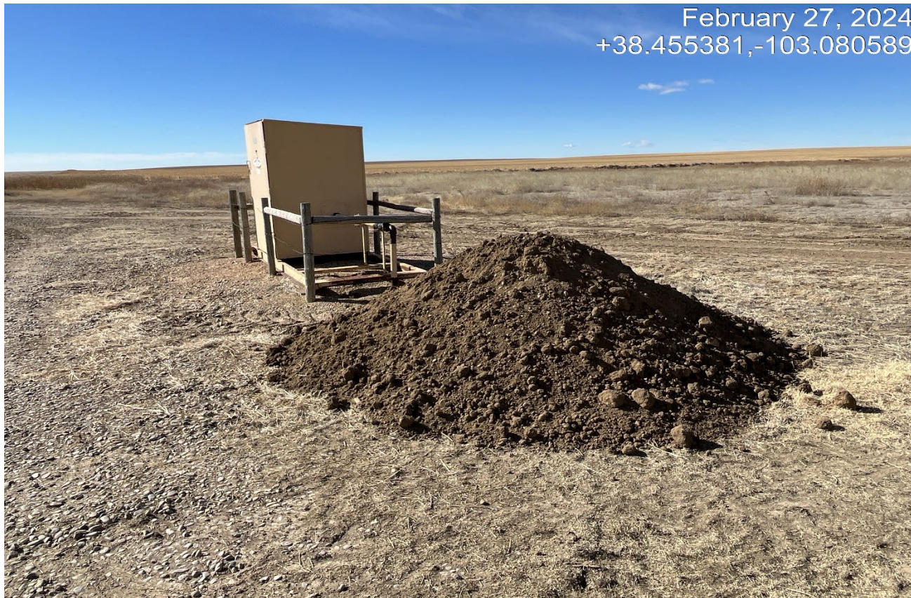
Photo 4. Facing southwest at the meter shed. This pile of soil contains impacted soils with a hydrocarbon odor. This pile needs to be properly disposed.
