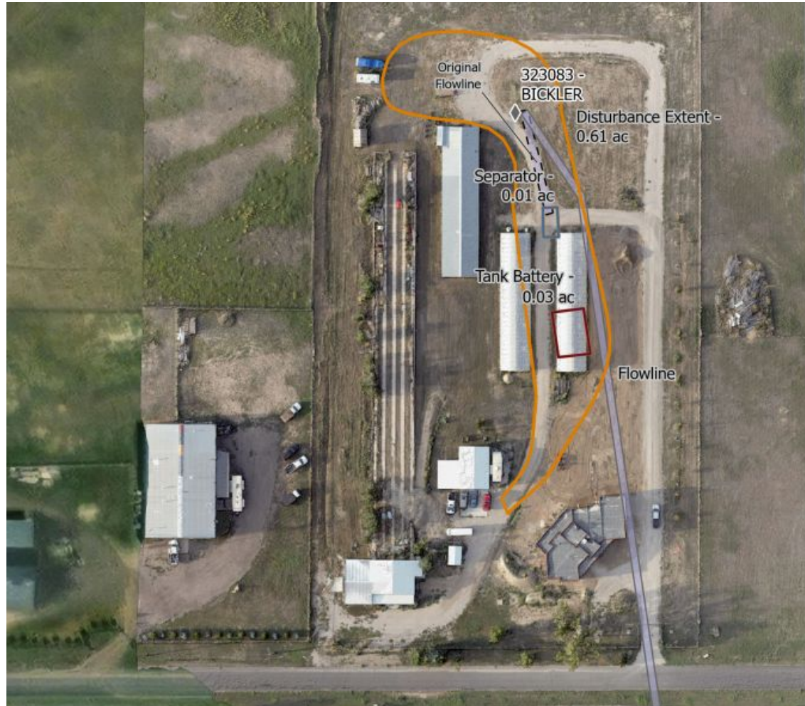
Photo 2. Aerial imagery from 2022 after plugging and abandonment operations. Imagery illustrates the surface owner has built over portions of the tank battery and well location. This imagery was submitted within the Form 4 Final Reclamation Complete Notice.
