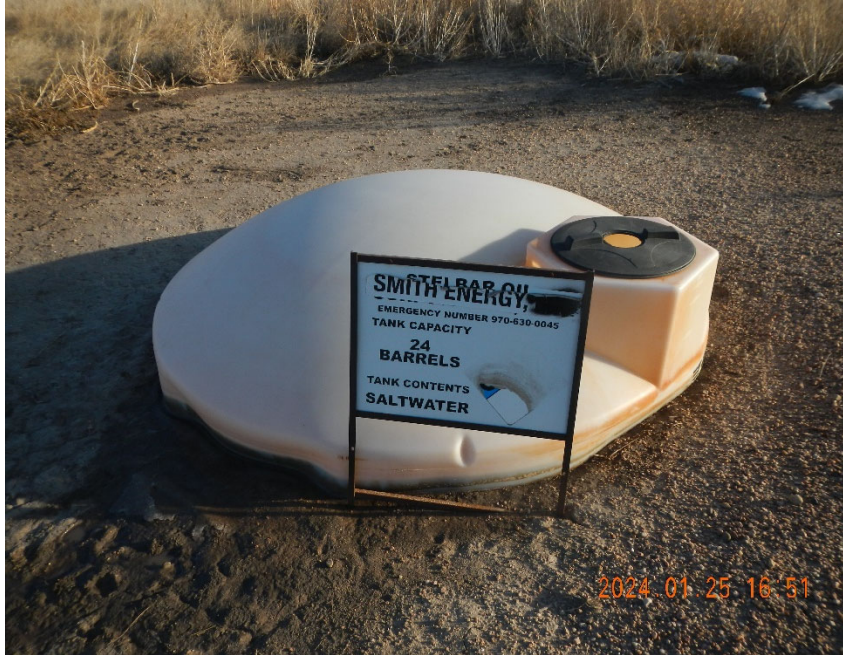
7. Produced water tank. Note hatch is missing plug.
