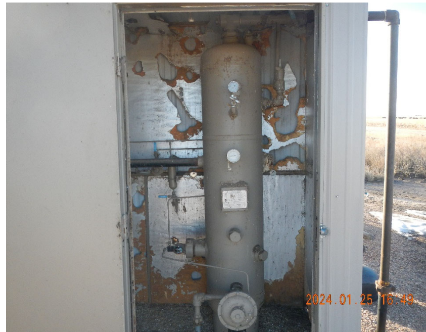
6. Vertical separator inside separator shed.
