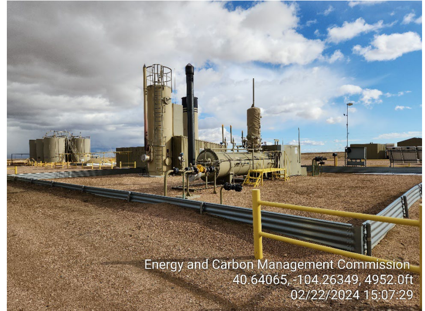
Photo 6 – Separator and Heater Treater
