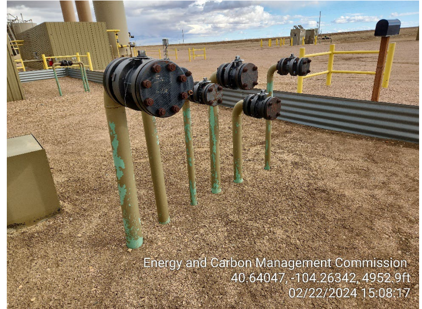
Photo 8 – Unmarked Risers
