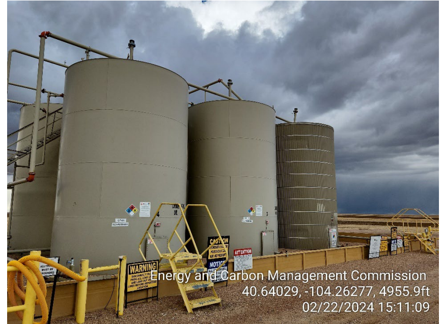
Photo 2 – Tank Battery
