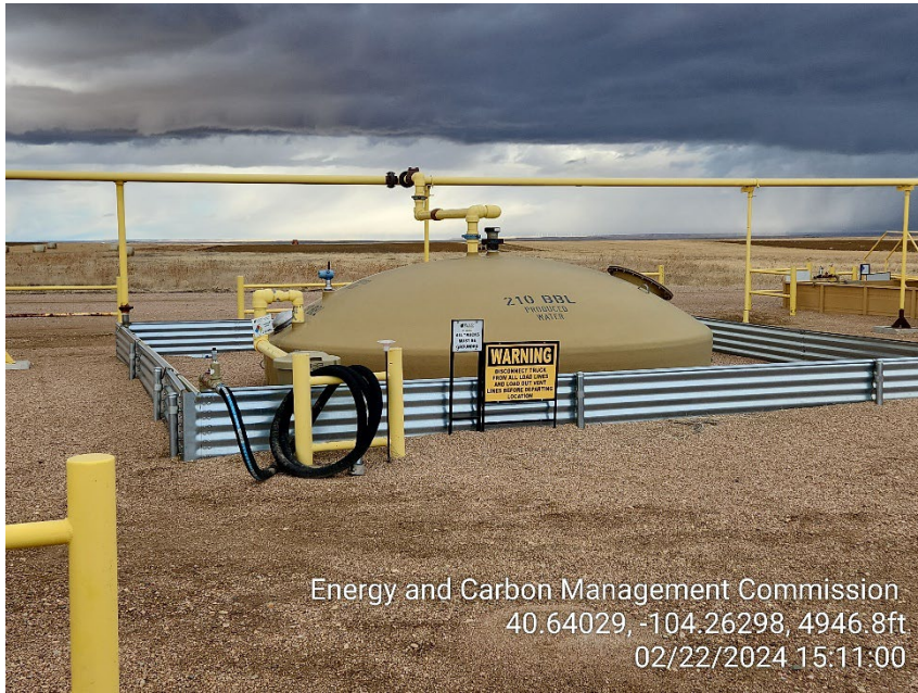
Photo 15 – Condensate Vault
