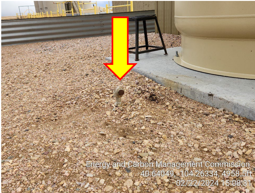
Photo 9 – Unmarked 1" Riser at Heater Treater
