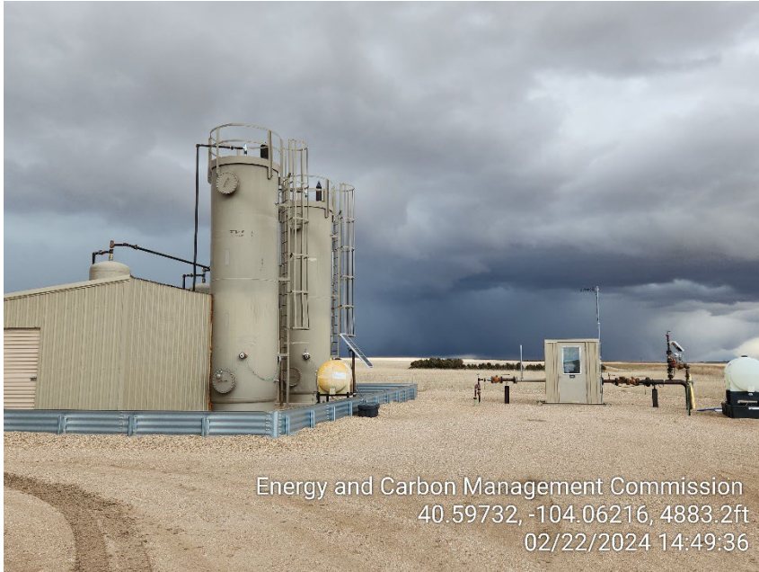
Photo 9 – Heater Treaters and Gas Meters
