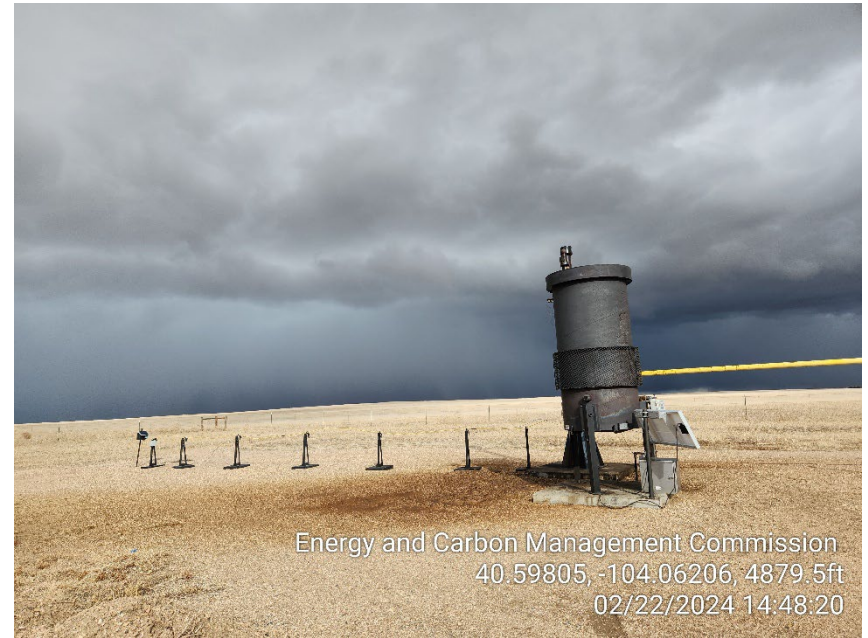
Photo 4 – Flare and ECD – Stained Soil
