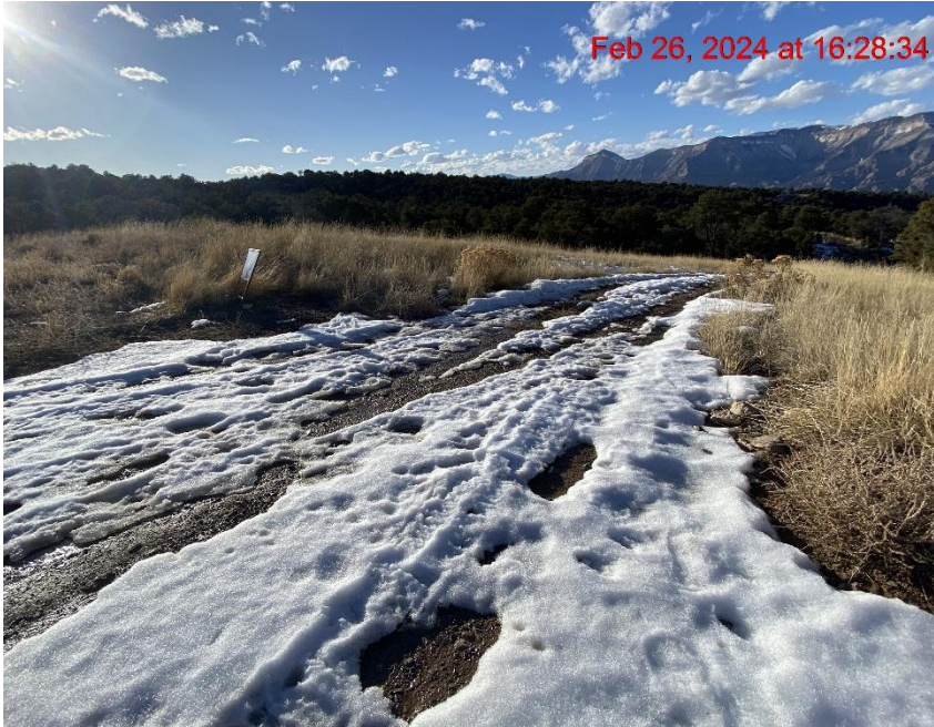
Insufficient Vehicle Tracking BMPs at Location Entrance/Exit – Photo #09552
