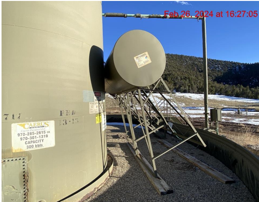
Methanol Tank Tipped Against Condensate Tank/General Safety – Photo #09548
