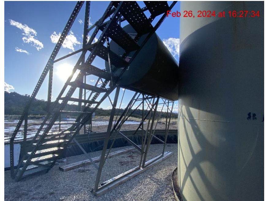
Methanol Tank Tipped Against Condensate Tank/General Safety – Photo #09549
