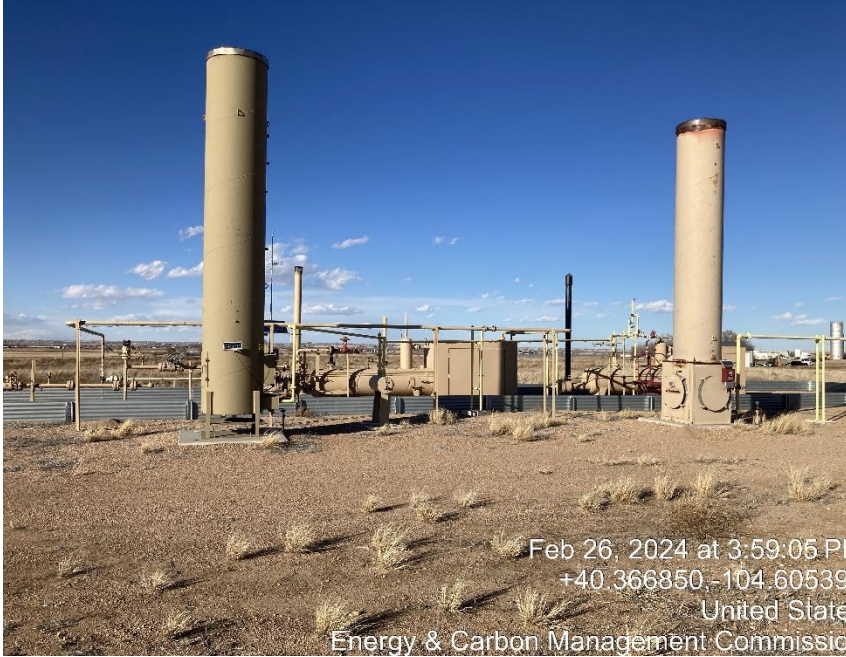
Photo 3 Separator/ECD
