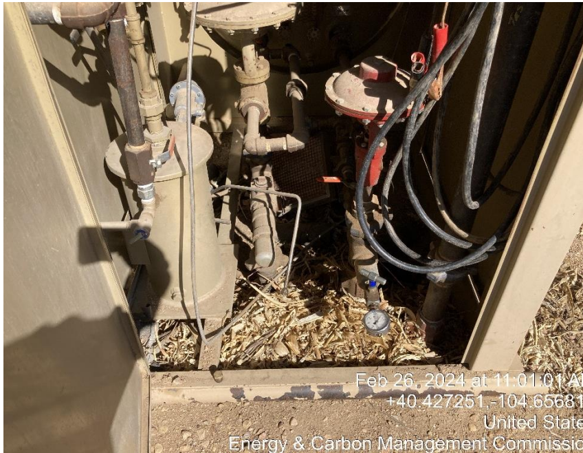
Photo 1 Separator house need to be cleaned fire hazard
