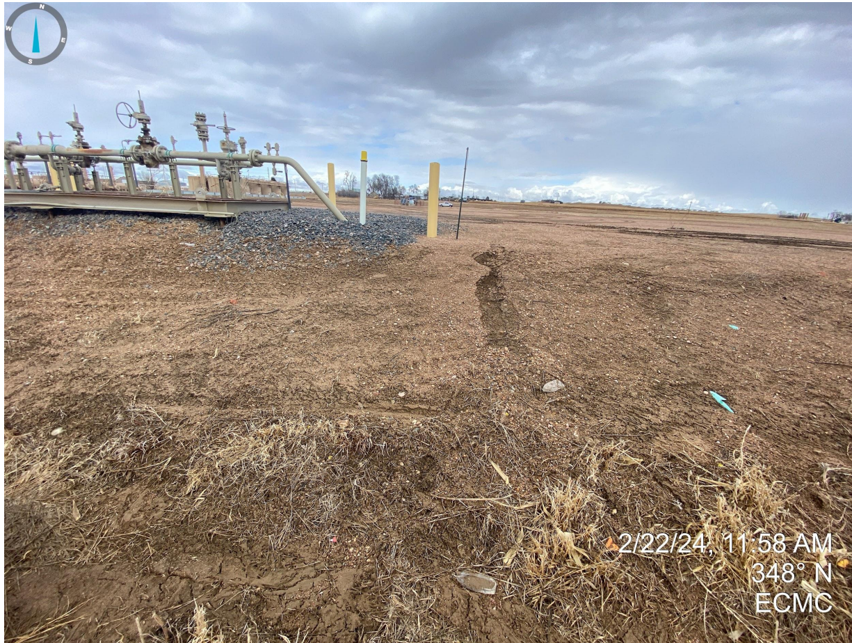
Photo 17. (Continued from Photo 16) Erosion degradation occurring on the southern side of the production areas.
