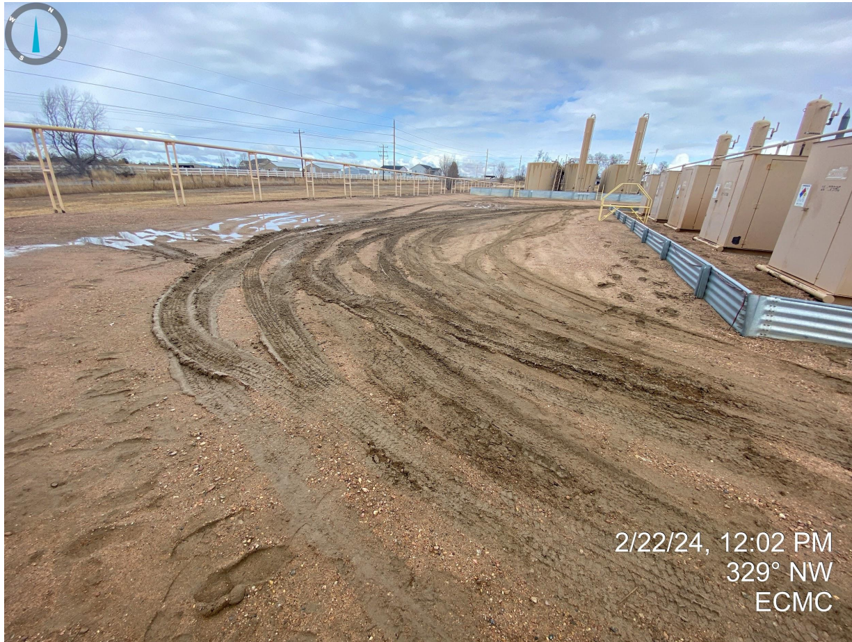
Photo 23. Unstabilized production areas require additional maintenance to prevent vehicle trackout.
