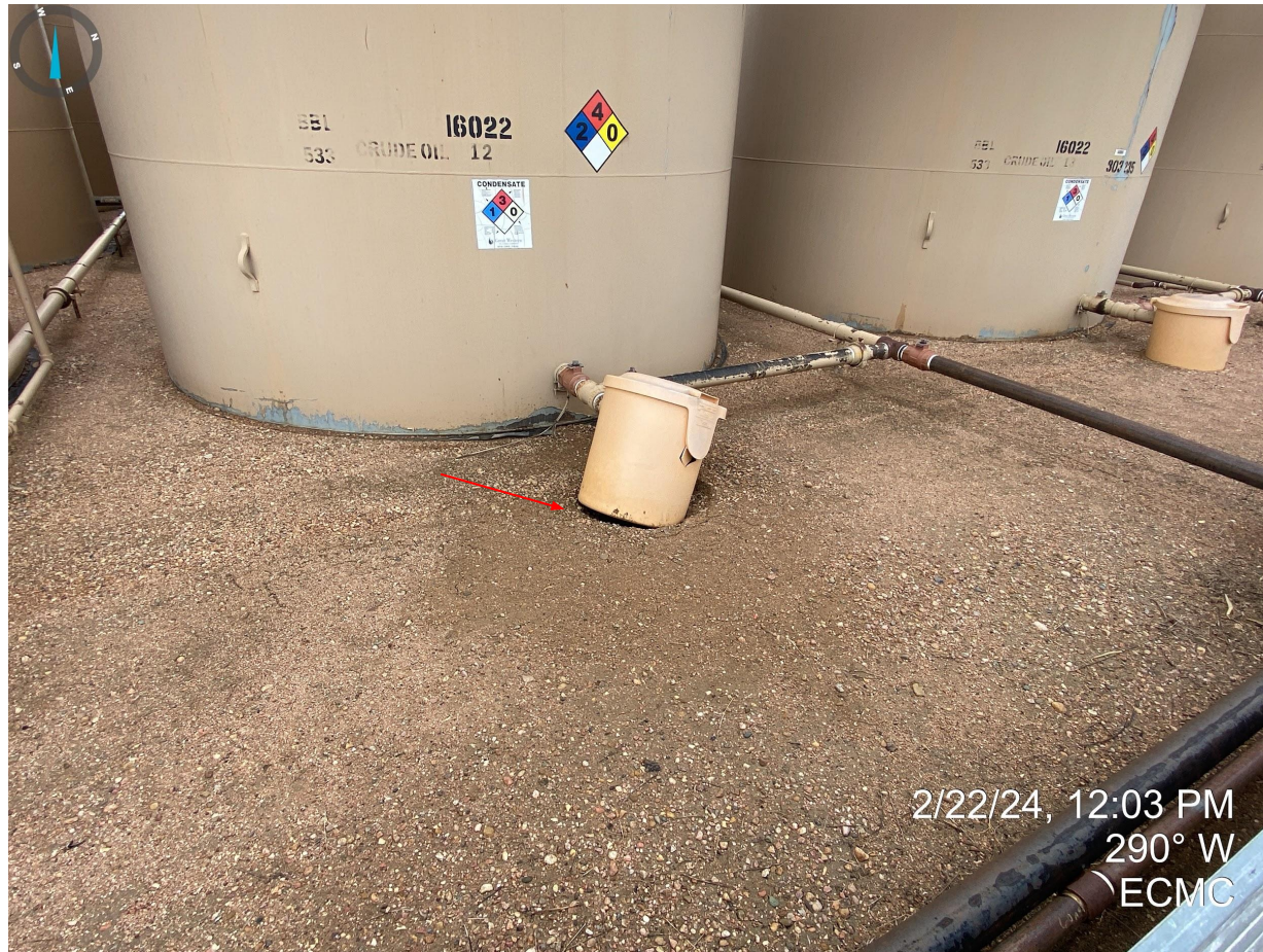
Photo 24. Subsidence located underneath loadout collection point.
