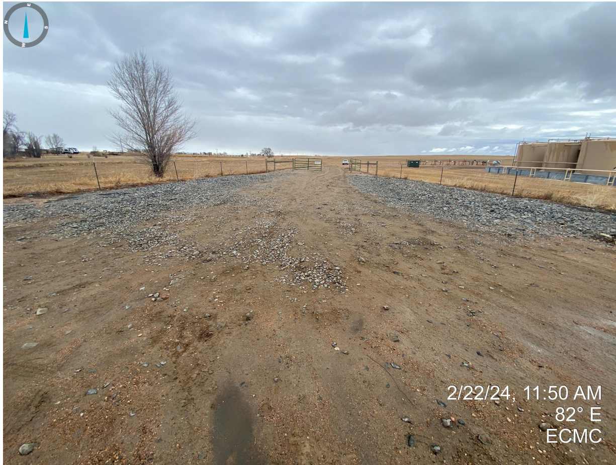
Photo 3. Vehicle track out pad requires maintenance.
