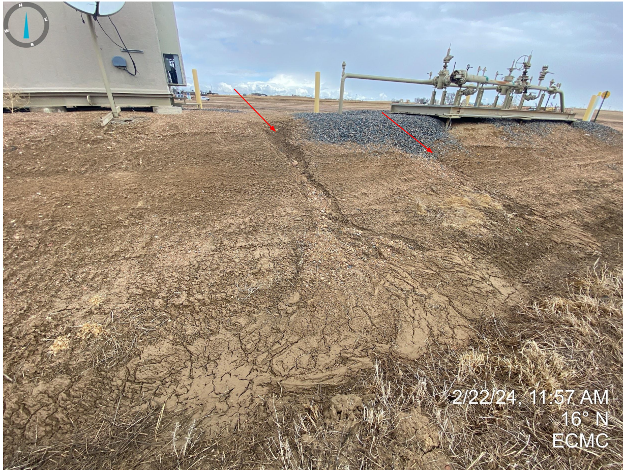
Photo 16. (Continued from Photo 15) Erosion degradation occurring on the southern side of the production areas.
