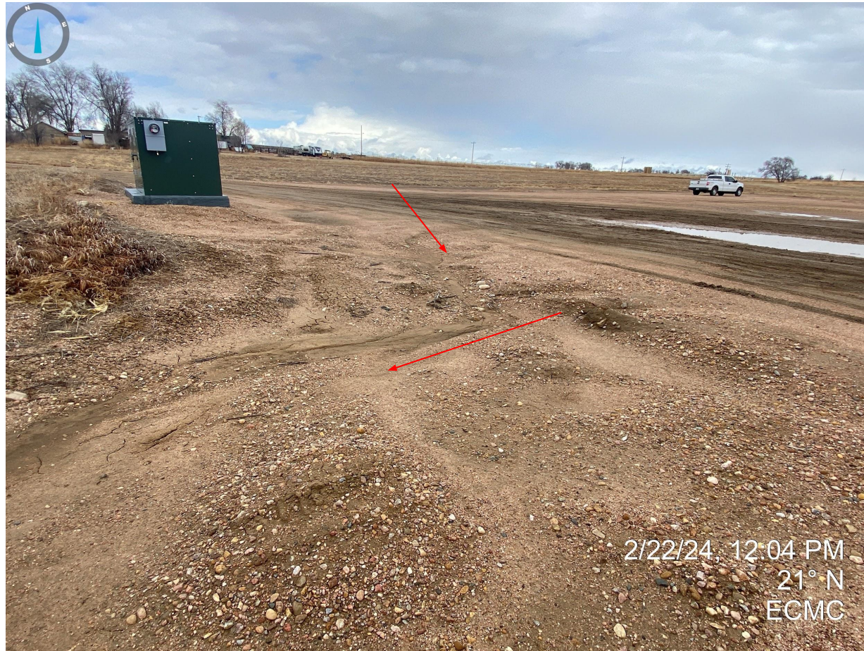
Photo 25. Erosion degradation located near the northern portion of the tank battery.
