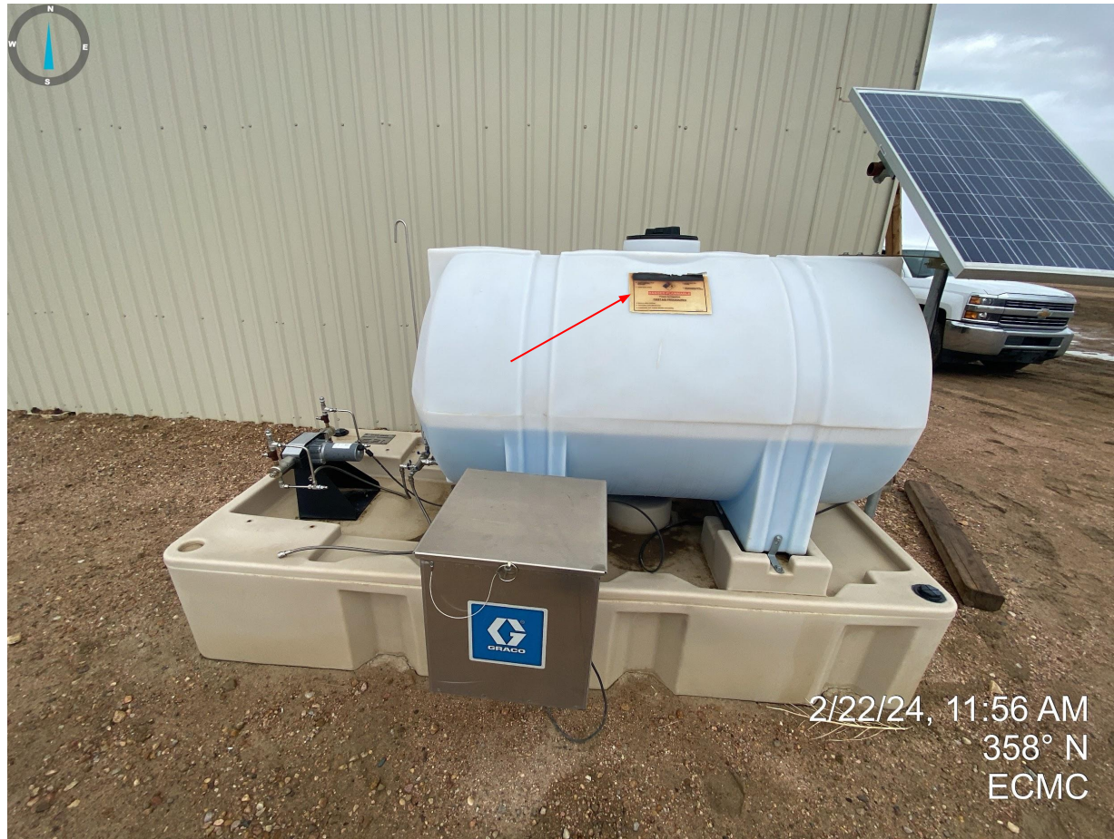
Photo 13. Tank labels are not legible (peeling, faded, cracked, etc).
