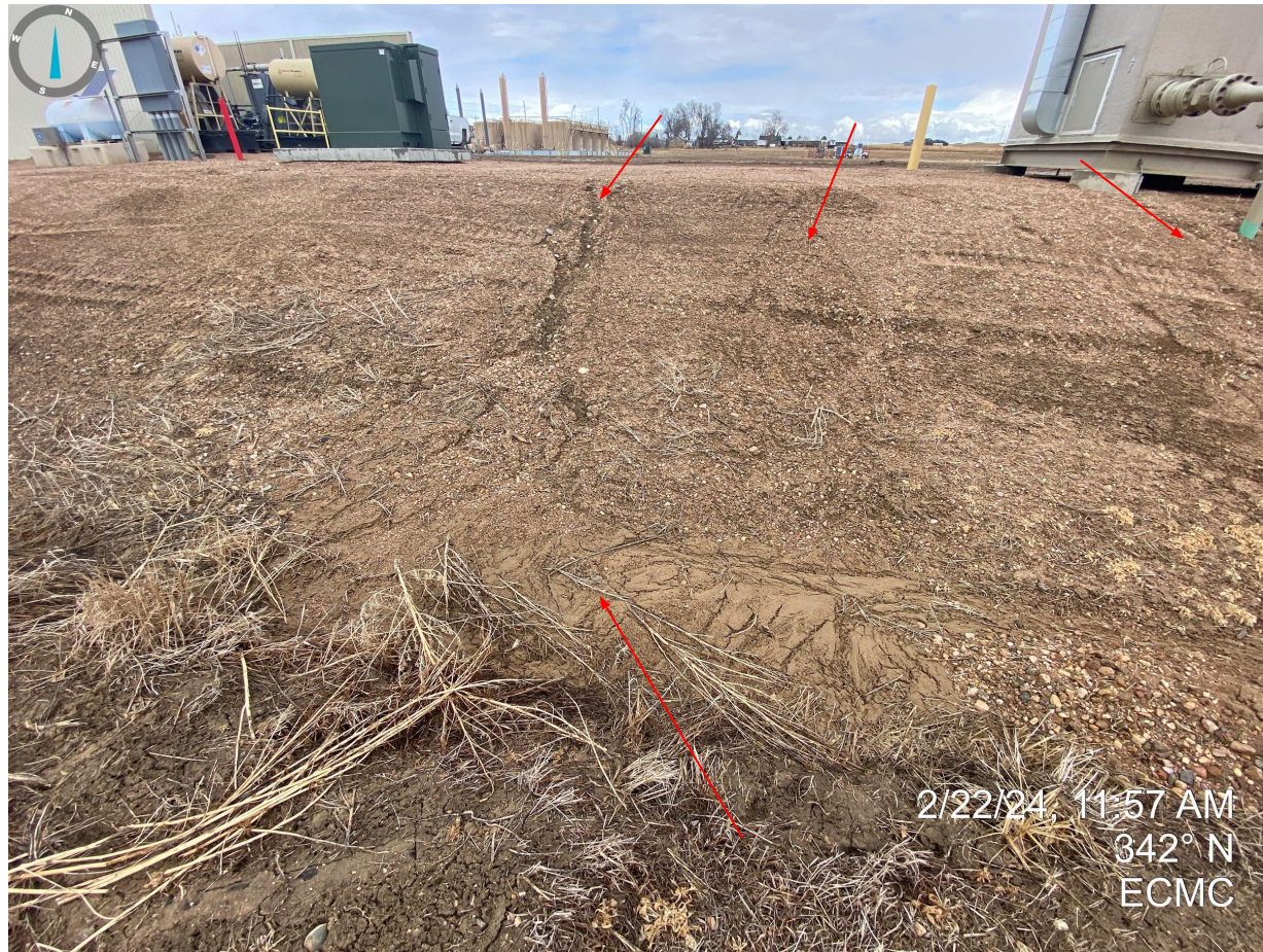
Photo 14. Erosion degradation occurring on the southern side of the production areas.
