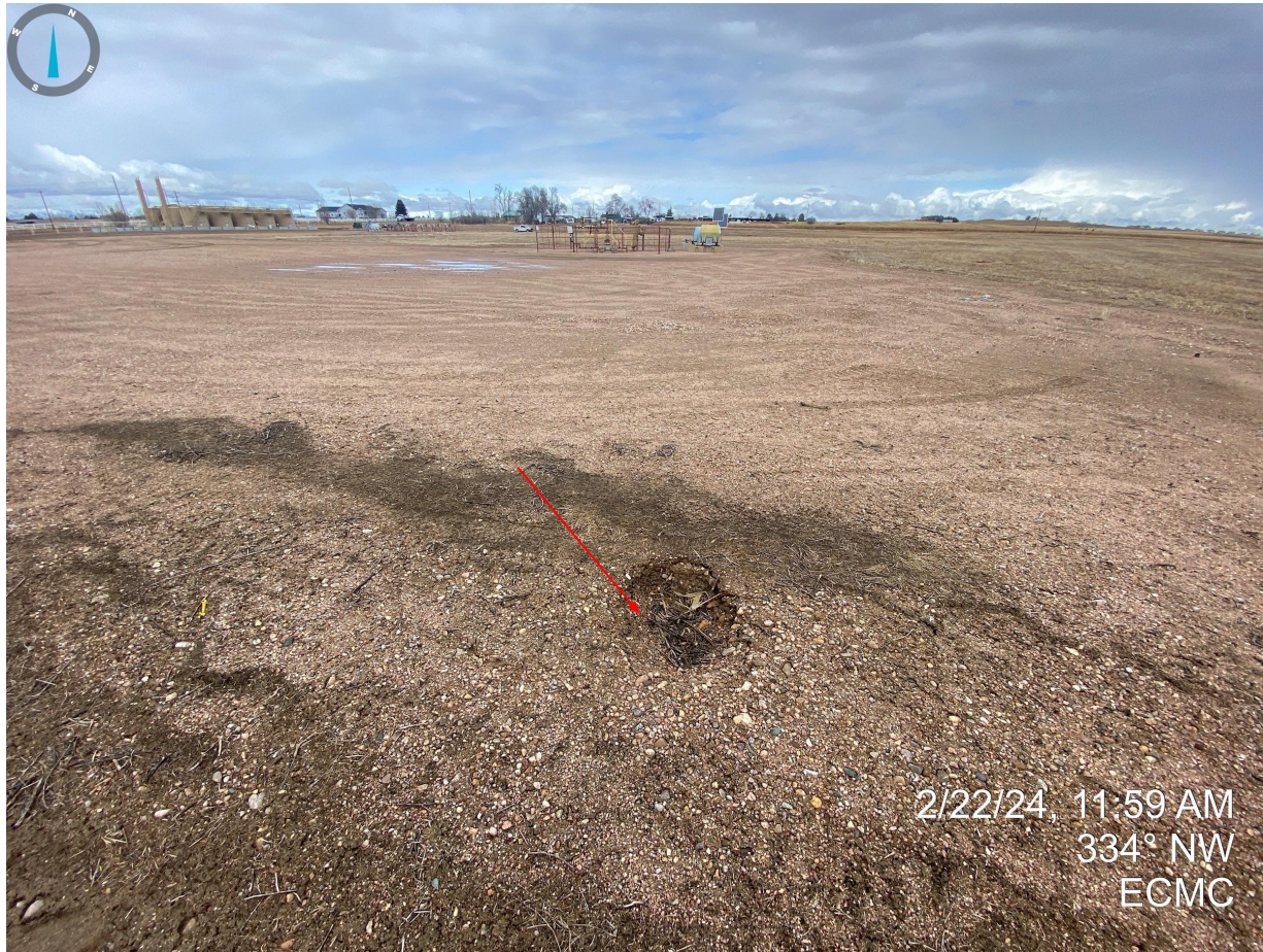
Photo 18. Hole/subsidence observed on the southeastern corner of the production areas.
