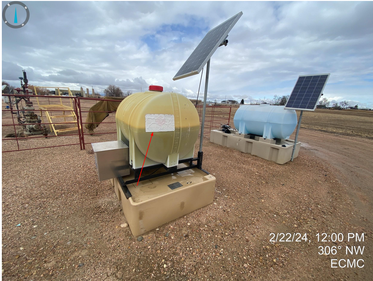
Photo 20. Tank labels are not legible (peeling, faded, cracked, etc).
