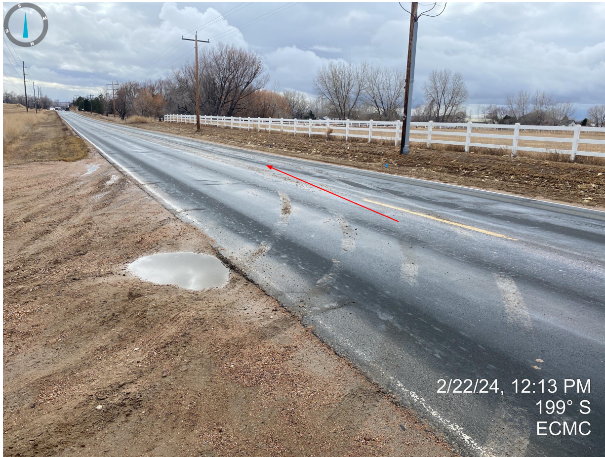
Photo 2. Taken from the location entrance; vehicle track out observed on County Road 19 (south bound lane).
