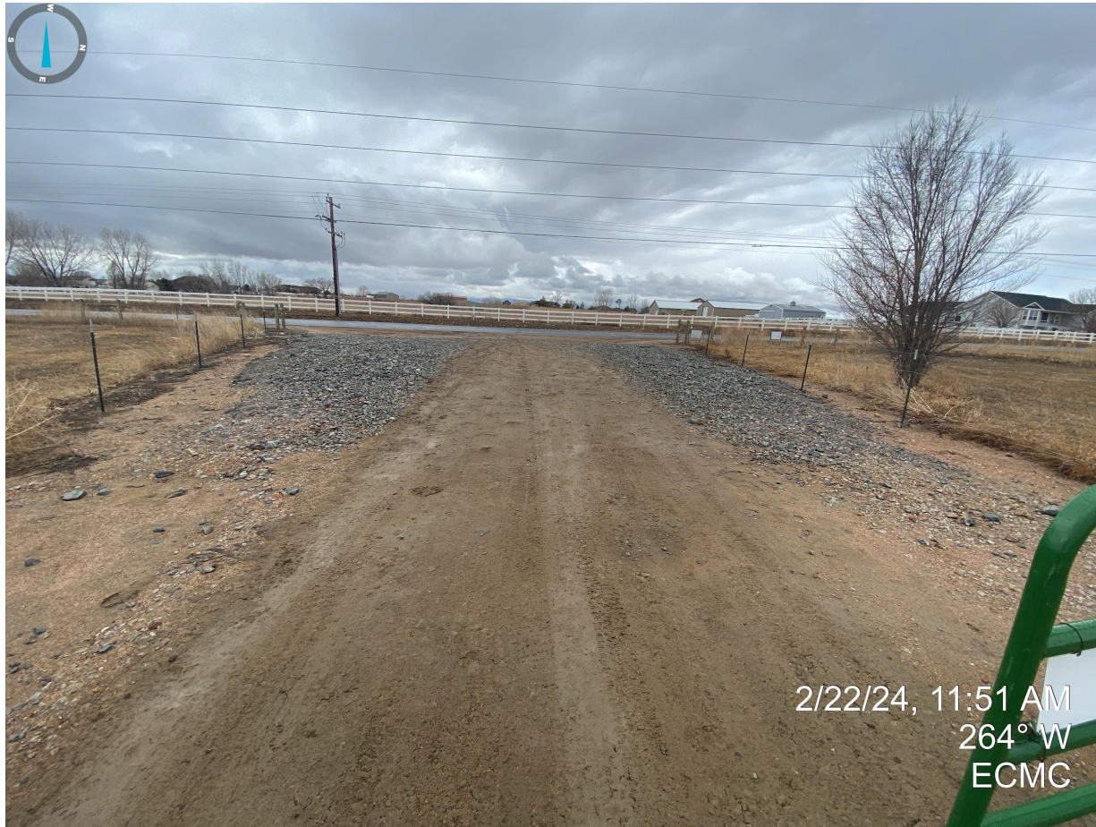
Photo 4. Vehicle track out pad requires maintenance.
