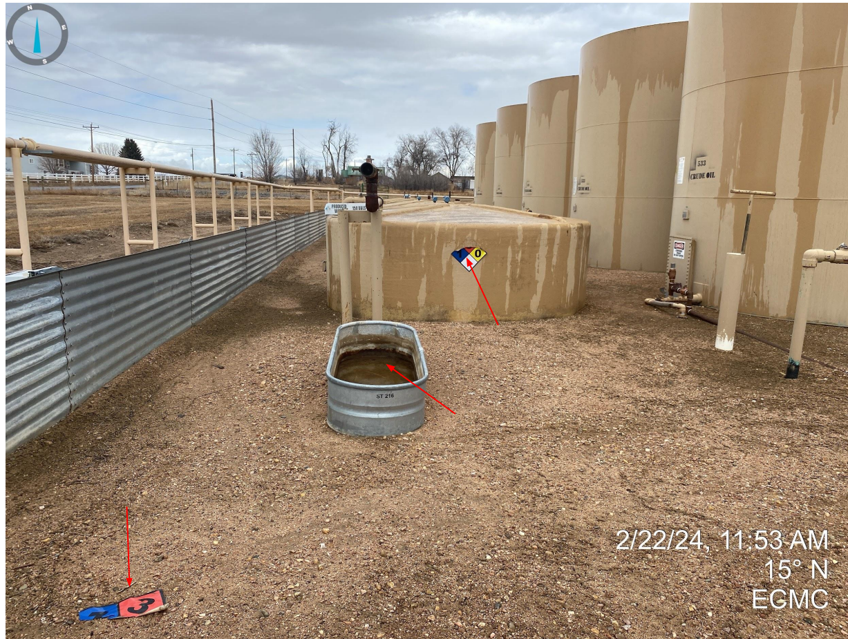
Photo 7. NFPA placard illegible at produced water tank and secondary containment without wildlife protection BMP.
