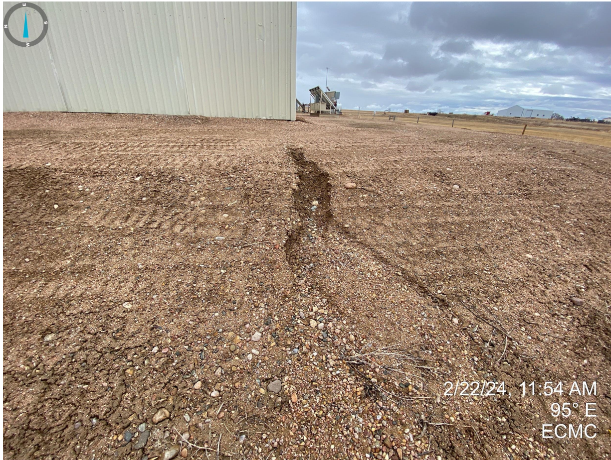
Photo 10. Erosion degradation occurring near the southwestern corner of the production areas.
