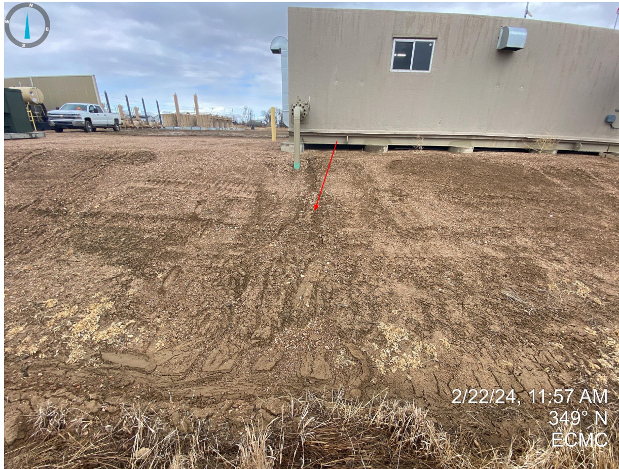
Photo 15. (Continued from Photo 14) Erosion degradation occurring on the southern side of the production areas.
