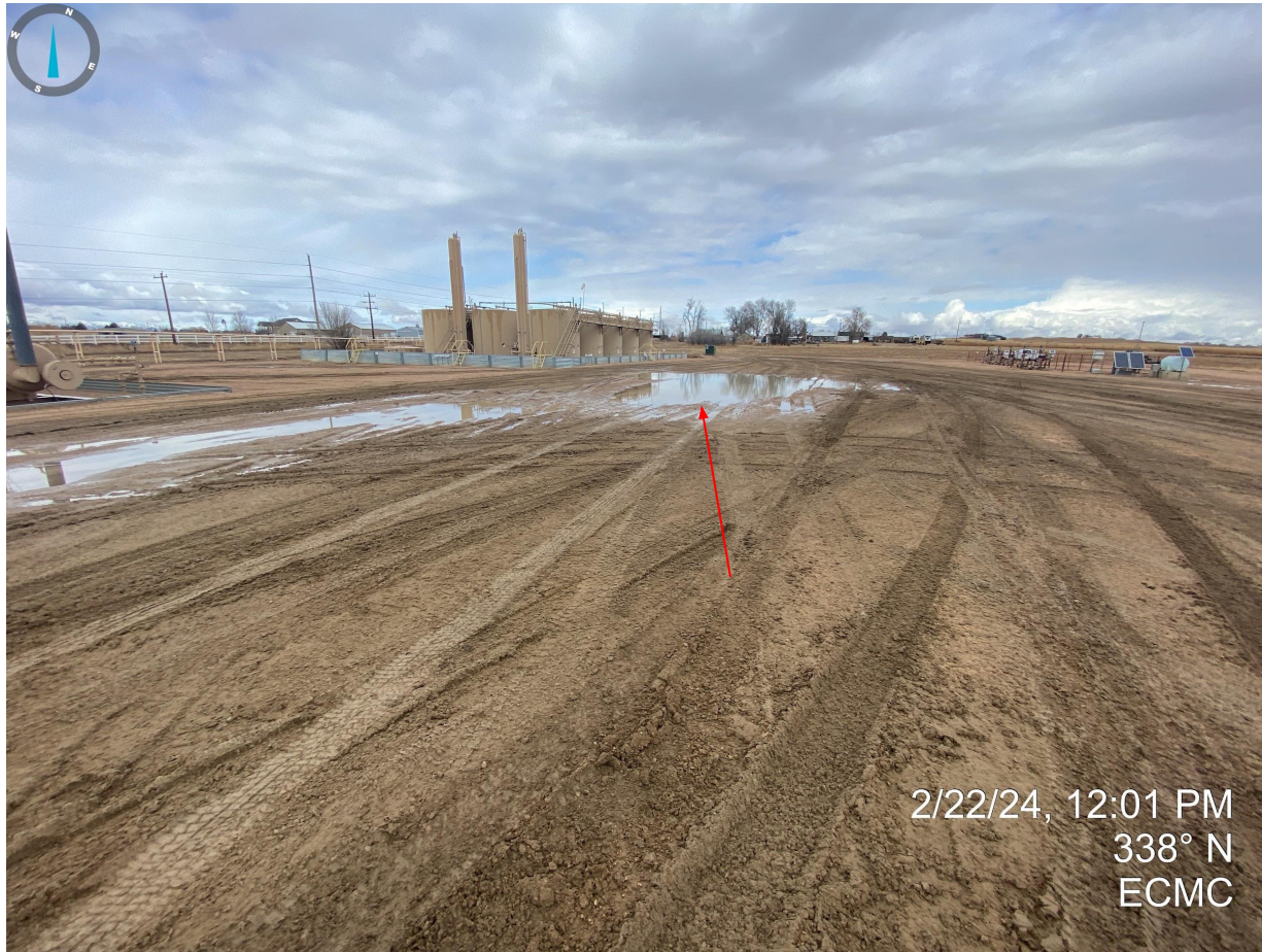
Photo 22. Unstabilized production areas require additional maintenance to prevent vehicle trackout.
