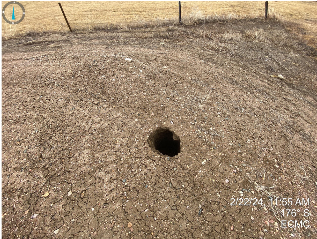
Photo 11. Hole/subsidence observed on the southwestern corner of the production areas.
