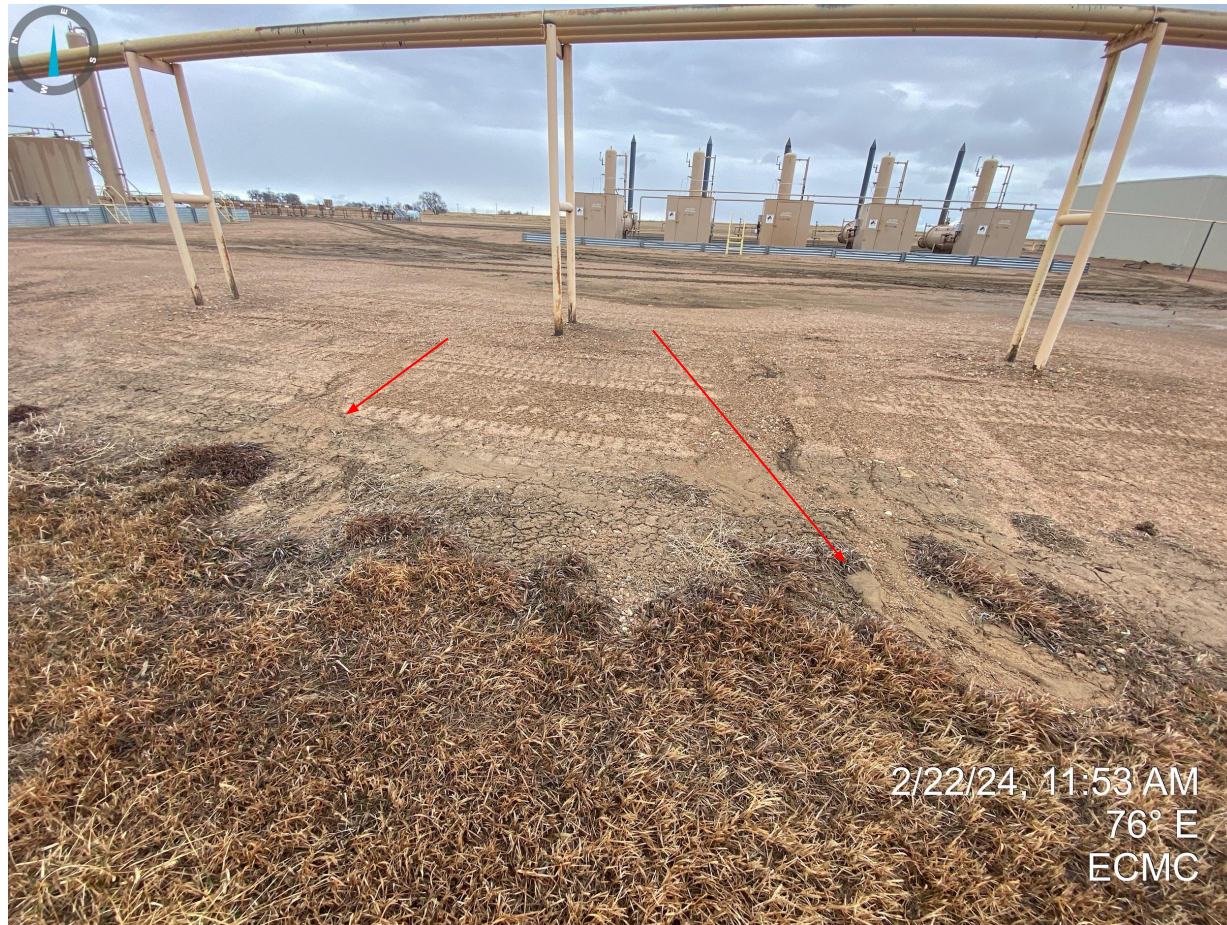
Photo 9. Erosion degradation occurring on the western side of the production areas.
