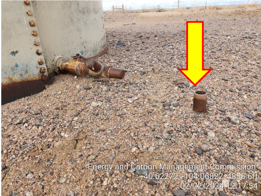
Photo 5 – Unmarked and Uncovered Riser
