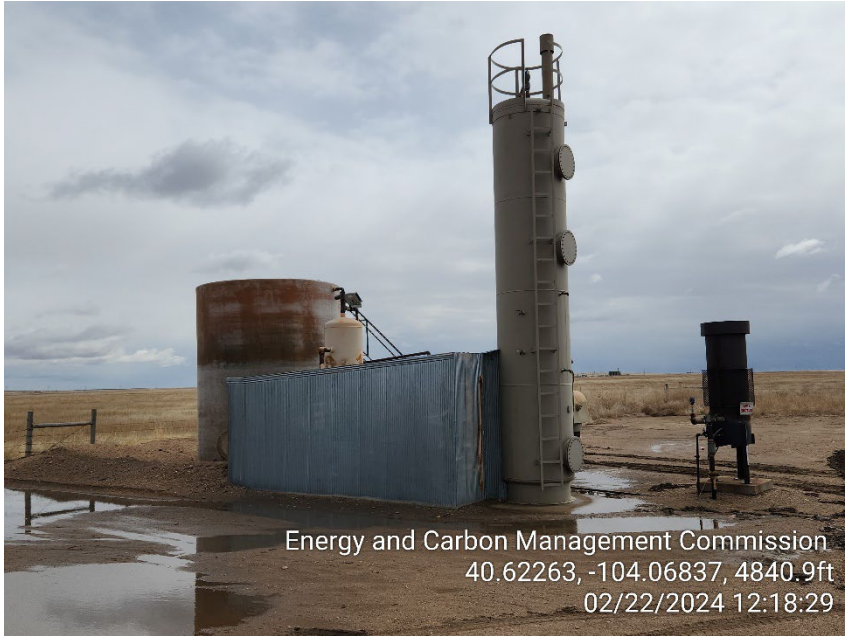
Photo 7 – Heater Treater and ECD
