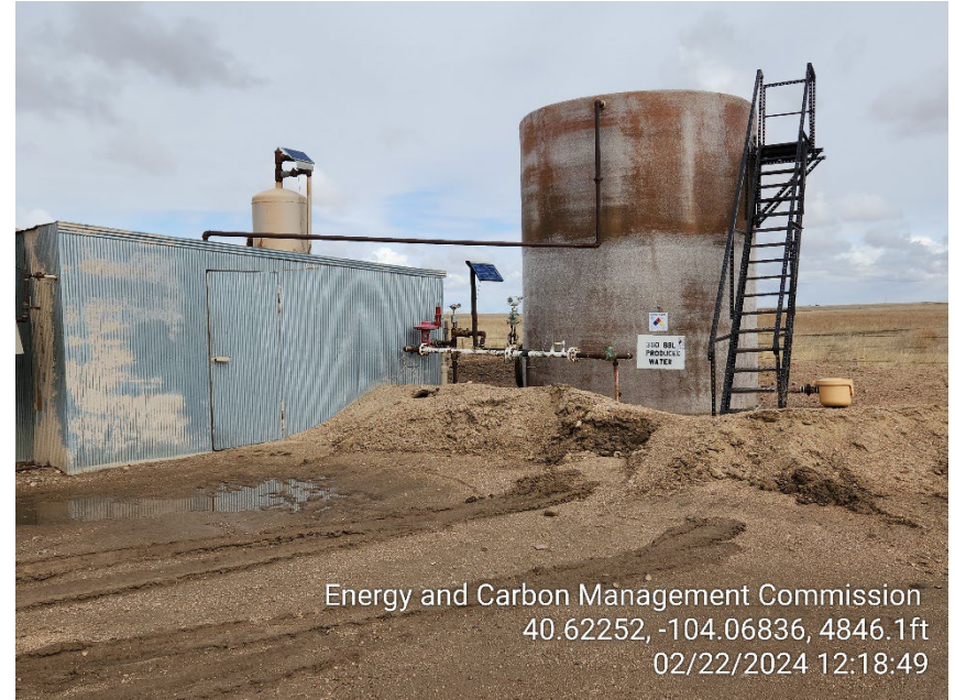
Photo 8 – Gas Meter and Produced Water Tank
