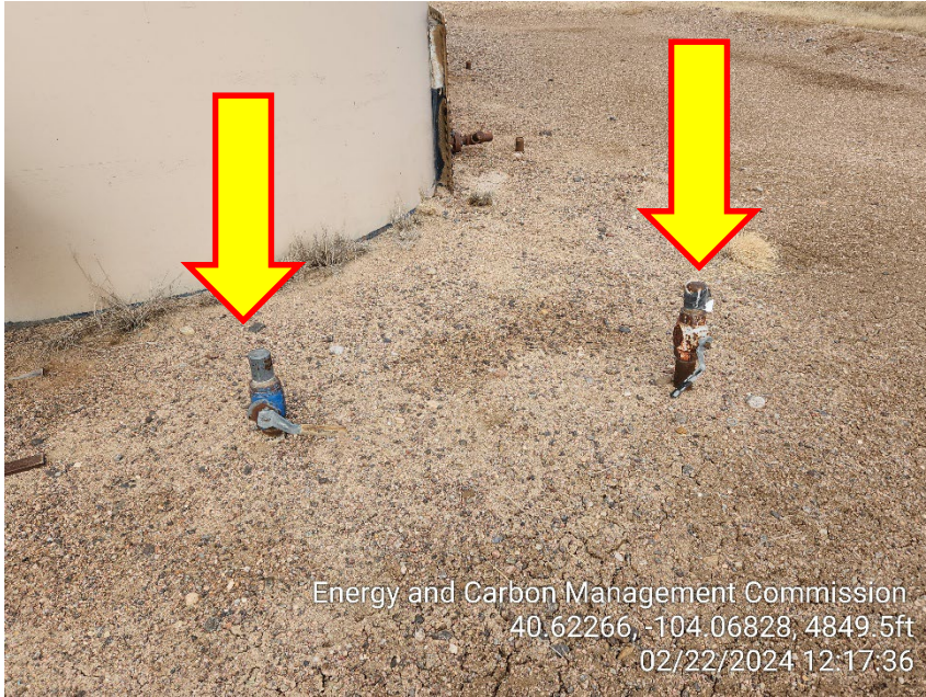
Photo 3 – Unmarked Risers
