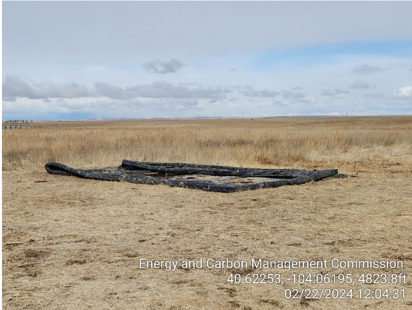
Photo 1 – Unused Secondary Containment
