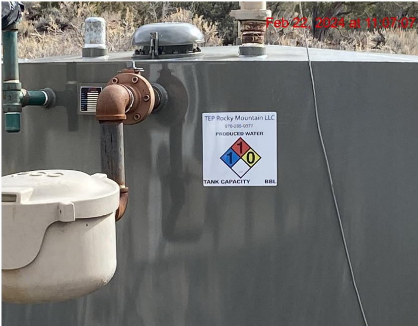
Label Missing Tank Capacity Information – Photo #09519
