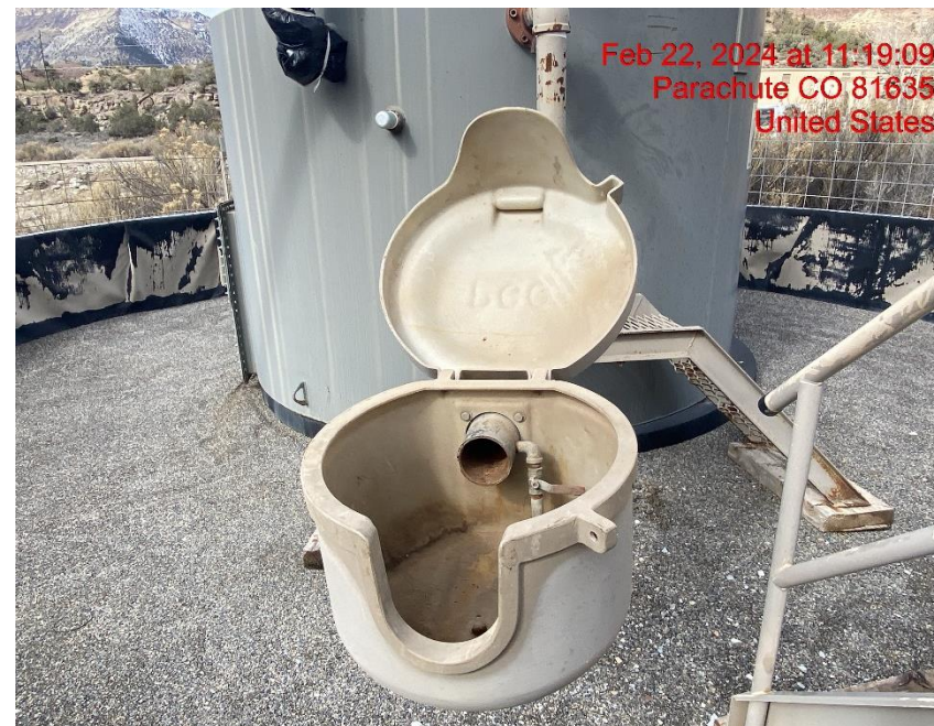
Open-Ended Load Line – Photo #09534
