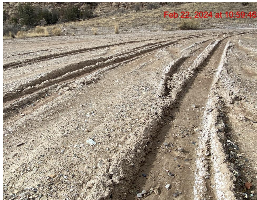
Lack of Stabilization – Photo #09508
