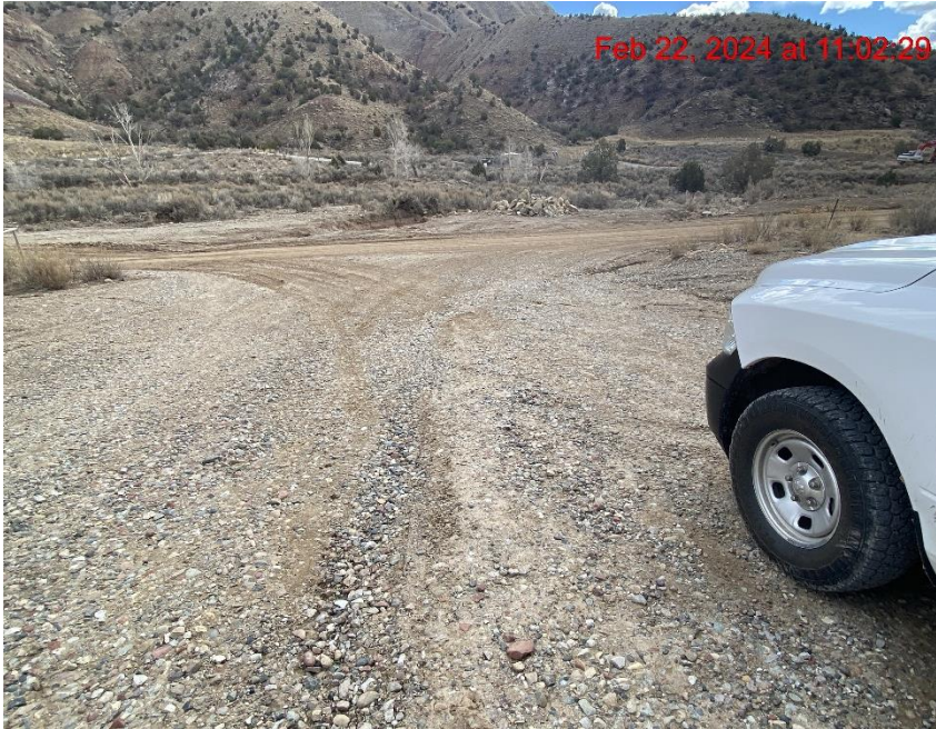
Insufficient Vehicle Tracking BMPs at Location Entrance/Exit – Photo #09513
