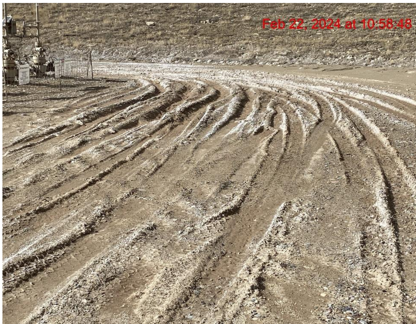
Lack of Stabilization – Photo #09506
