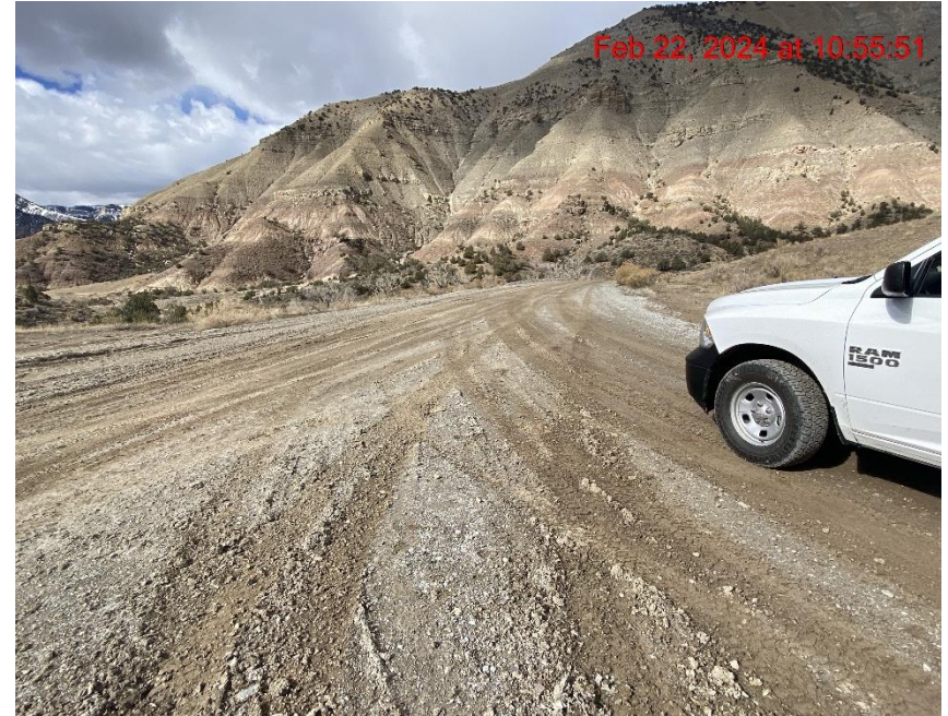
Insufficient Vehicle Tracking BMPs at Location Entrance/Exit – Photo #09502
