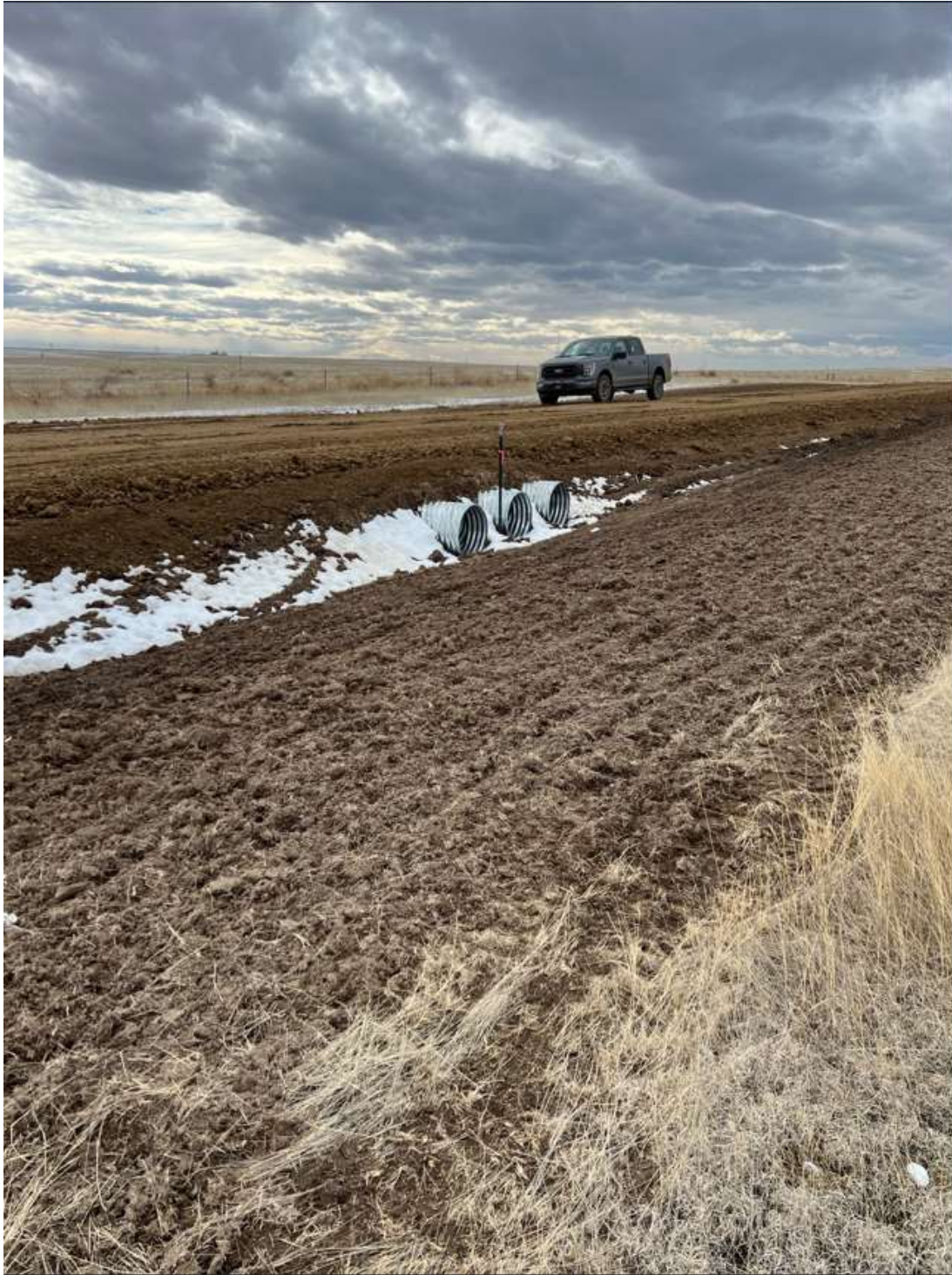
Photo 6. Taken near the west culvert crossing (north side). There was no further topsoil to salvage from this crossing, as we had already taken it out prior to setting culverts. Topsoil was not used as backfill for culverts. Excess fill material from pad was used as backfill.
