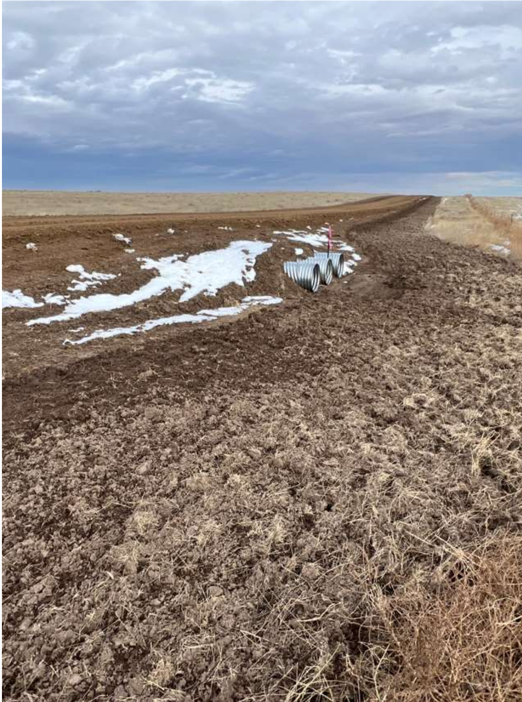
Photo 3. Taken near the west culvert crossing (south side). There was no further topsoil to salvage from this crossing, as we had already taken it out prior to setting culverts. Topsoil was not used as backfill for culverts. Excess fill material from pad was used as backfill.
