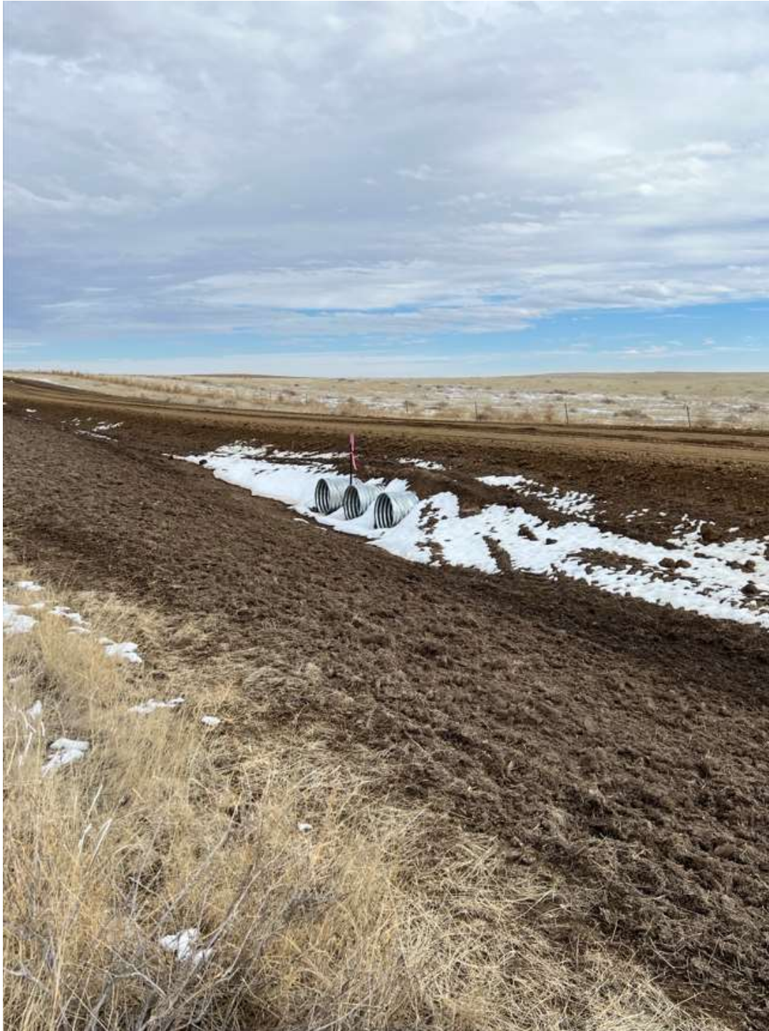
Photo 2. Taken near the west culvert crossing (north side). There was no further topsoil to salvage from this crossing, as we had already taken it out prior to setting culverts. Topsoil was not used as backfill for culverts. Excess fill material from pad was used as backfill.
