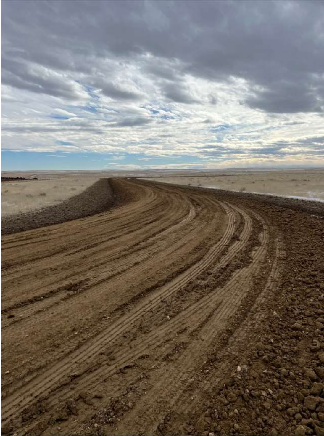
Photo 7. Taken near the entrance to the drilling pad and the access road. Before the first inspection 3" of topsoil was stripped from the access road and pushed to the side to be used in the v-ditches and slopes of the road. After the first inspection an additional 3" of topsoil was stripped from the road and used to topsoil the cut slopes, fill slopes, berms, and detention pond on pad.
