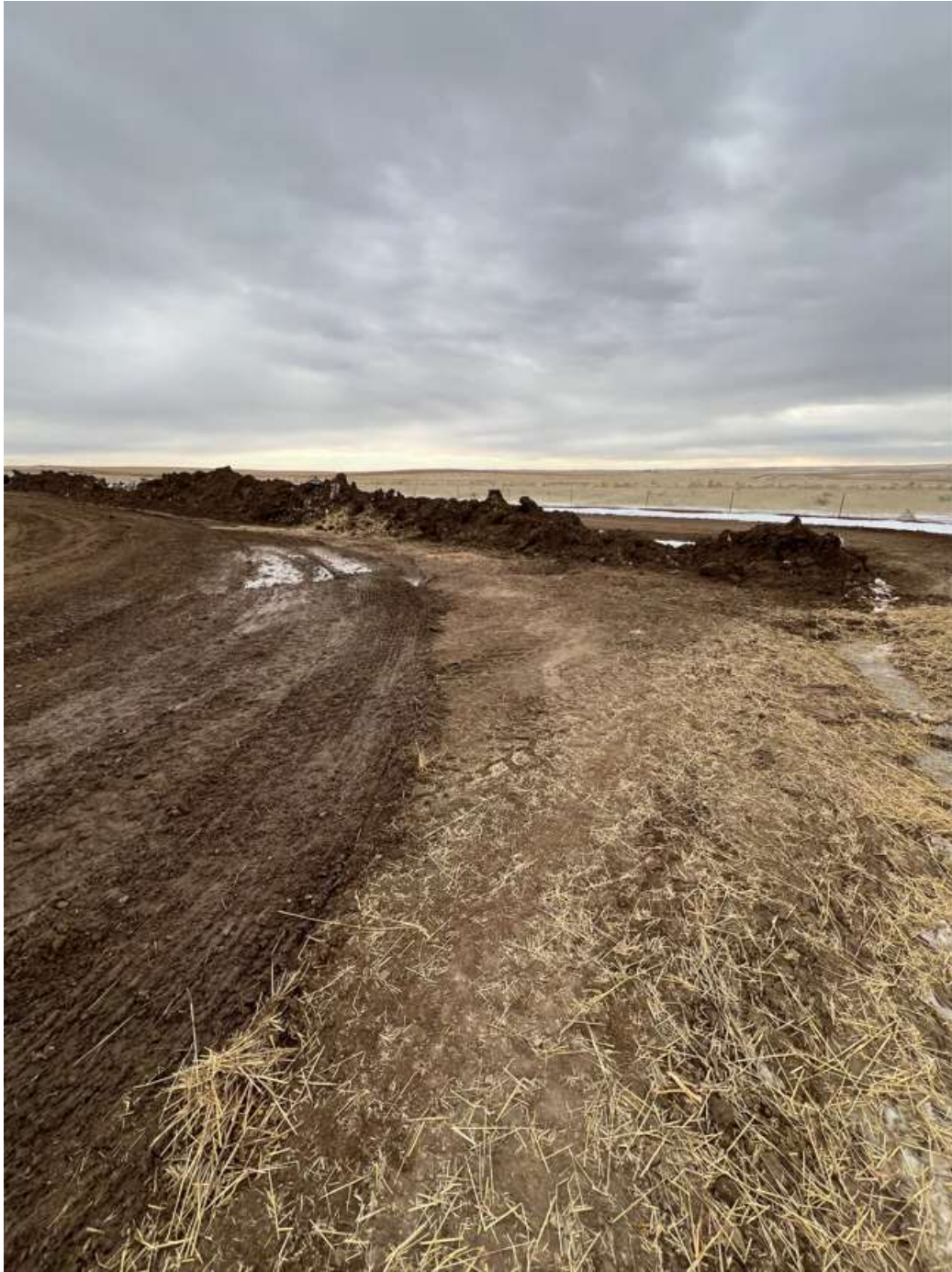
Photo 22. Erosion degradation and sediment transport has been fixed in the southwest corner of the drilling pad.
