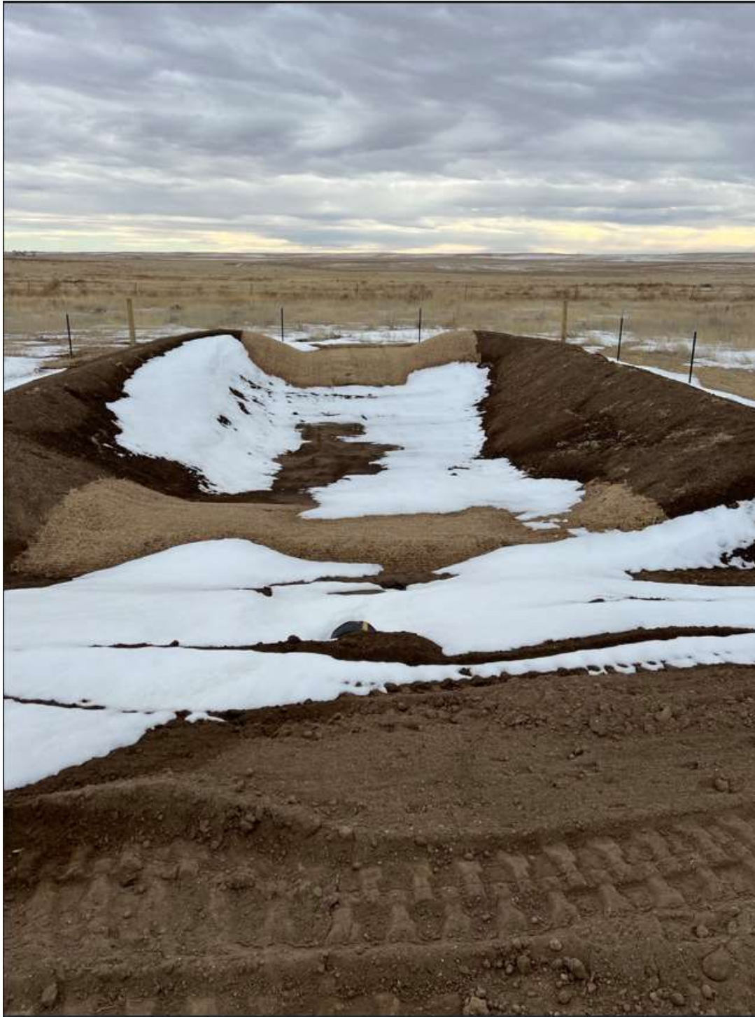
Photo 13. Northeast sediment trap is still under construction. Will be completed once weather permits.
