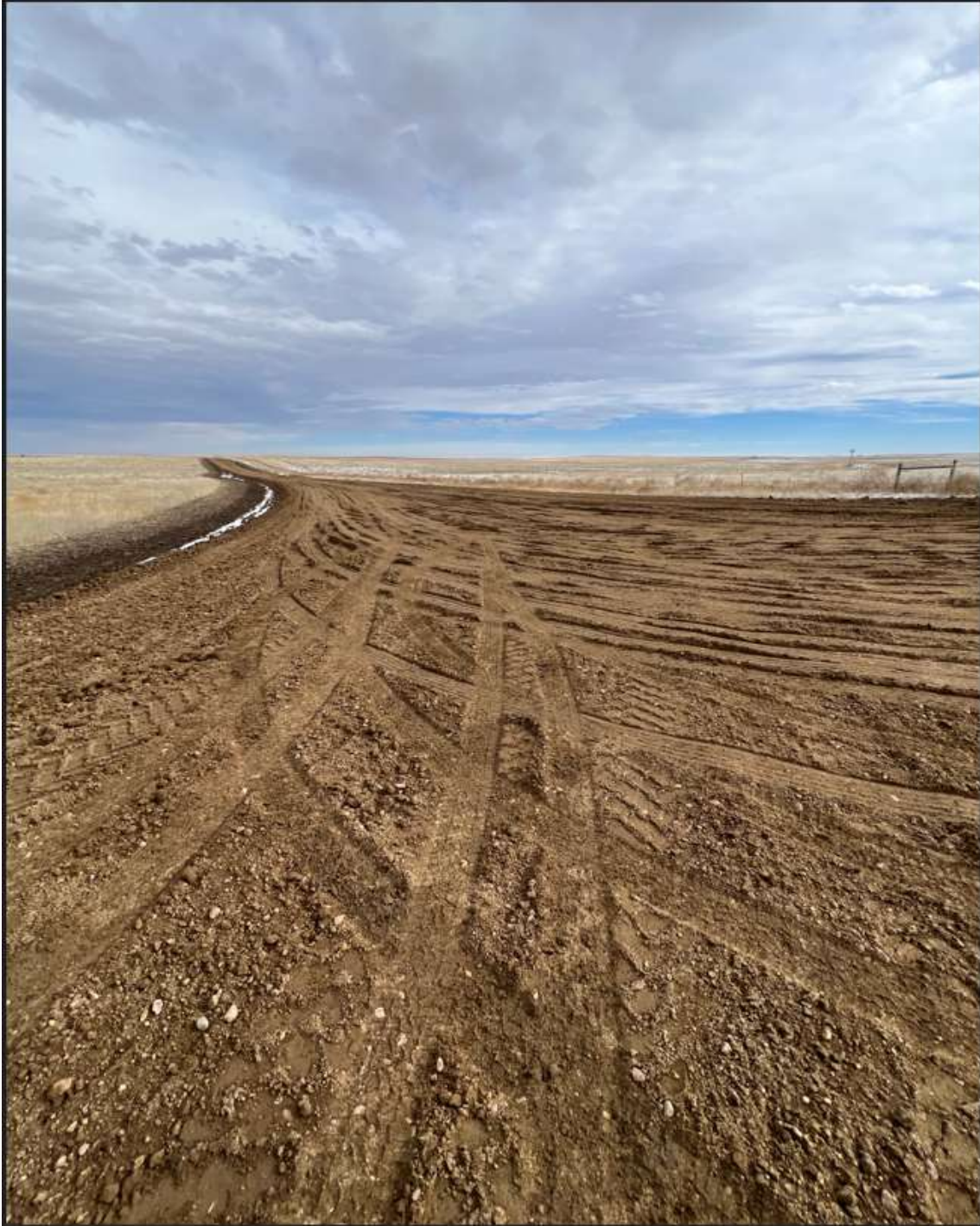
Photo 1. Taken from the start (west end) of the access road. Before the first inspection 3" of topsoil was stripped from the access road and pushed to the side to be used in the v-ditches and slopes of the road. After the first inspection an additional 3" of topsoil was stripped from the road and used to topsoil the cut slopes, fill slopes, berms, and detention pond on pad.
