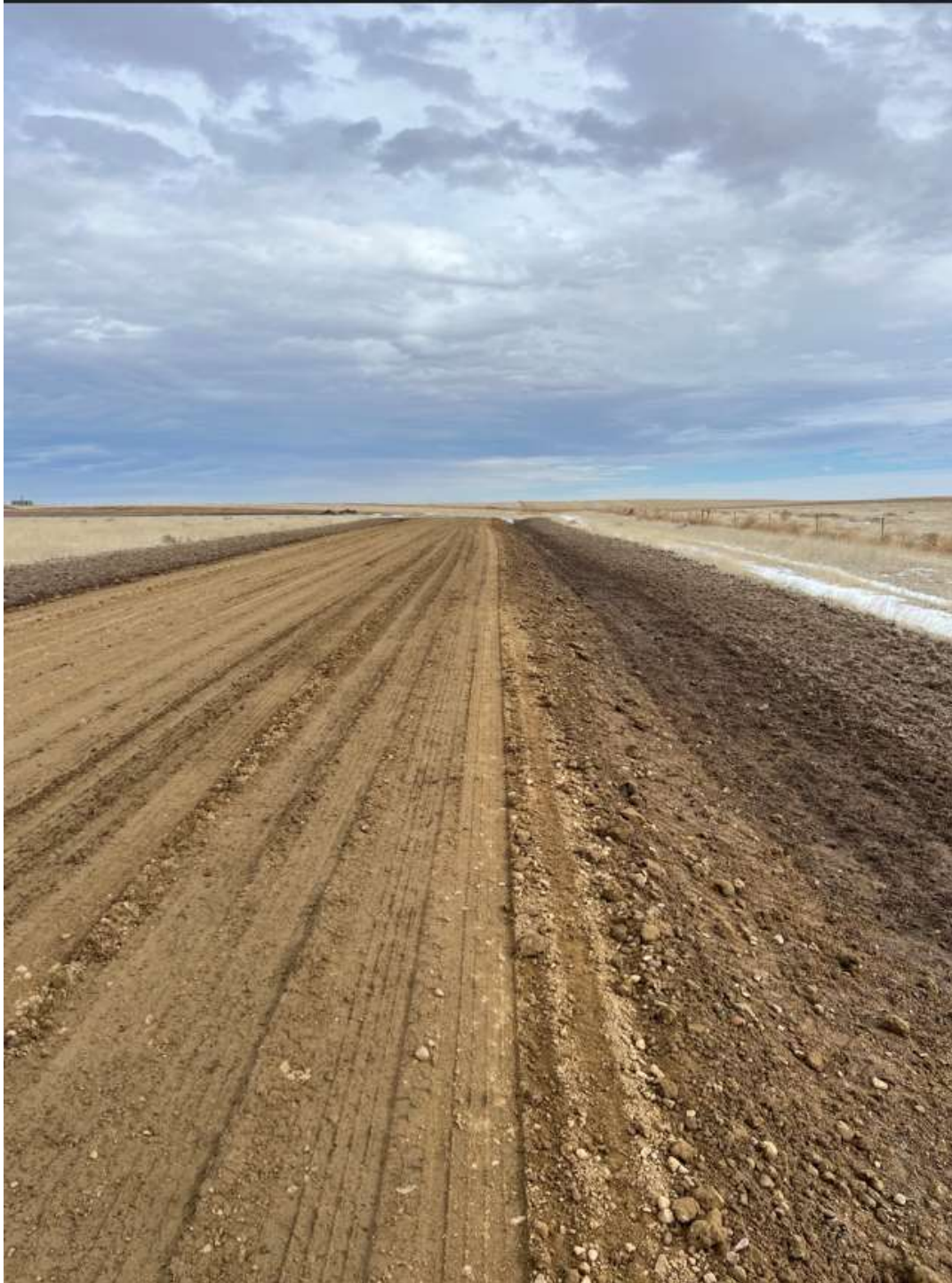
Photo 4. Taken from the middle portion (between the two culverts) of the access road. Before the first inspection 3" of topsoil was stripped from the access road and pushed to the side to be used in the v-ditches and slopes of the road. After the first inspection an additional 3" of topsoil was stripped from the road and used to topsoil the cut slopes, fill slopes, berms, and detention pond on pad.
