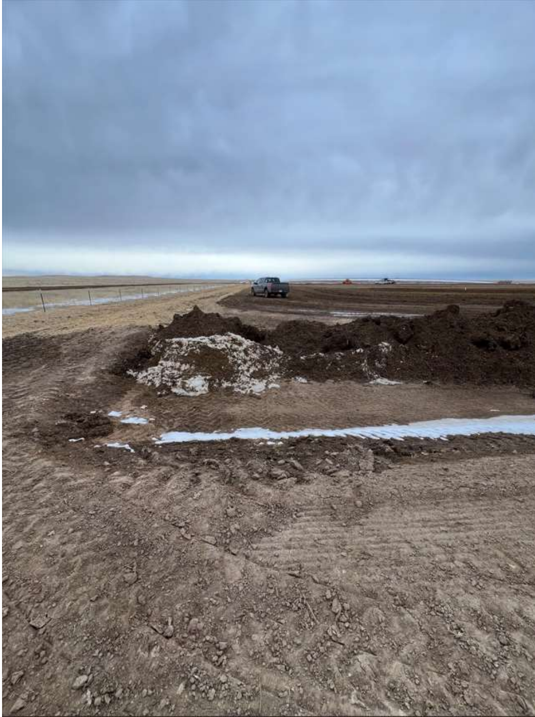
Photo 21. Erosion degradation has been fixed in the southwest corner of the drilling pad.
