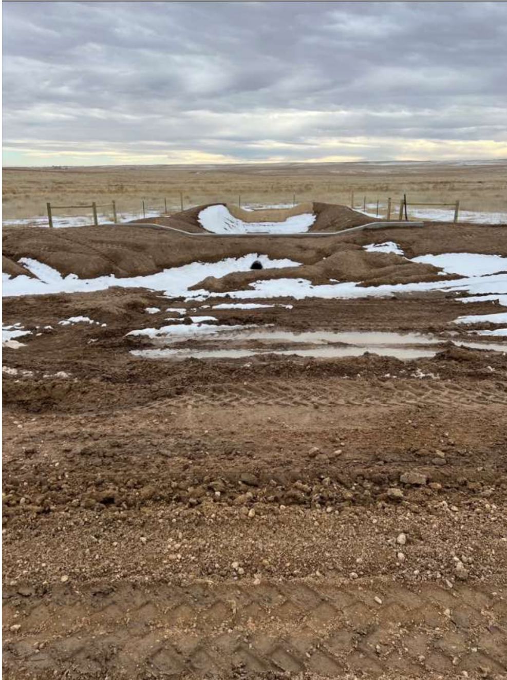
Photo 18. Erosion degradation has been fixed near the southern sediment trap. The southern sediment trap is still being constructed and will be completed once weather permits.
