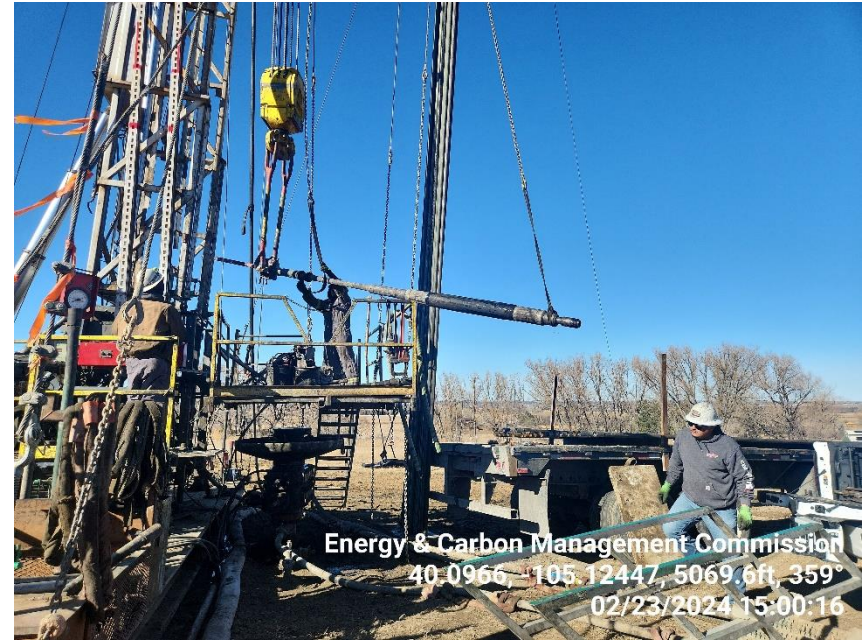
Photo 8 Packer out of the hole.
