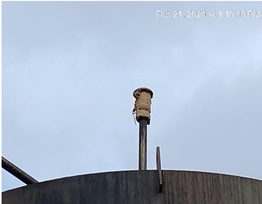
Oily waste covering relief valves
