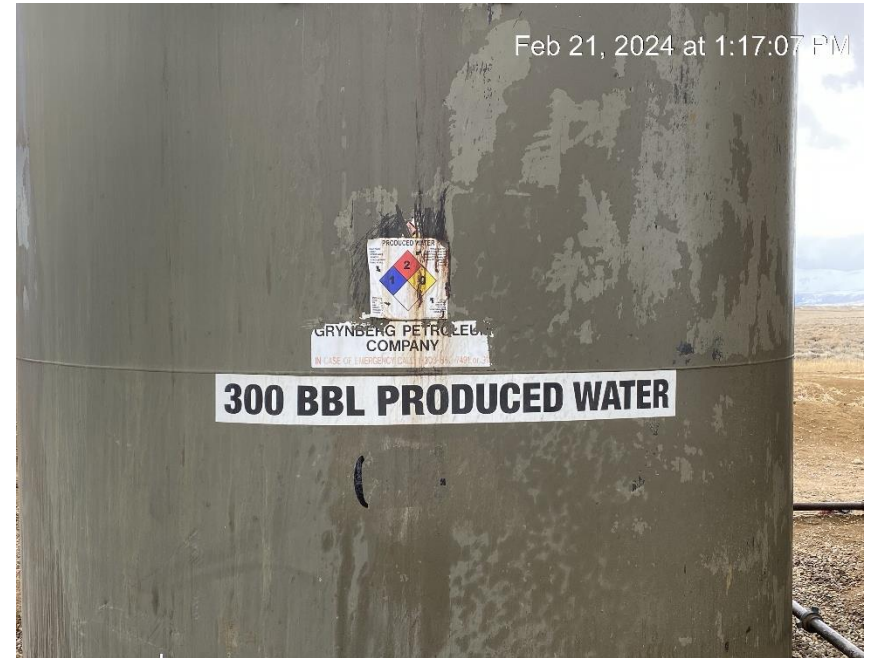
Tank labels missing required information
