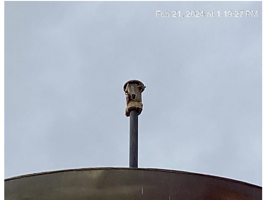
Oily waste covering relief valves
