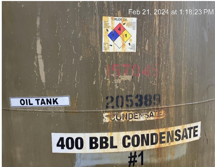
Tank labels missing required information
