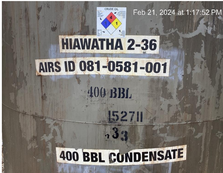
Tank labels missing required information
