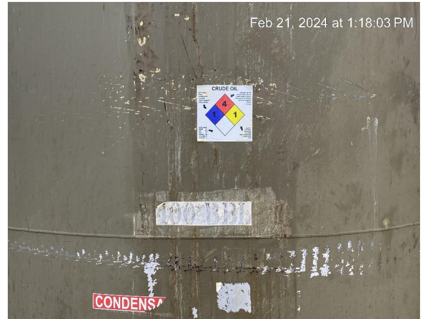
Tank labels missing required information
