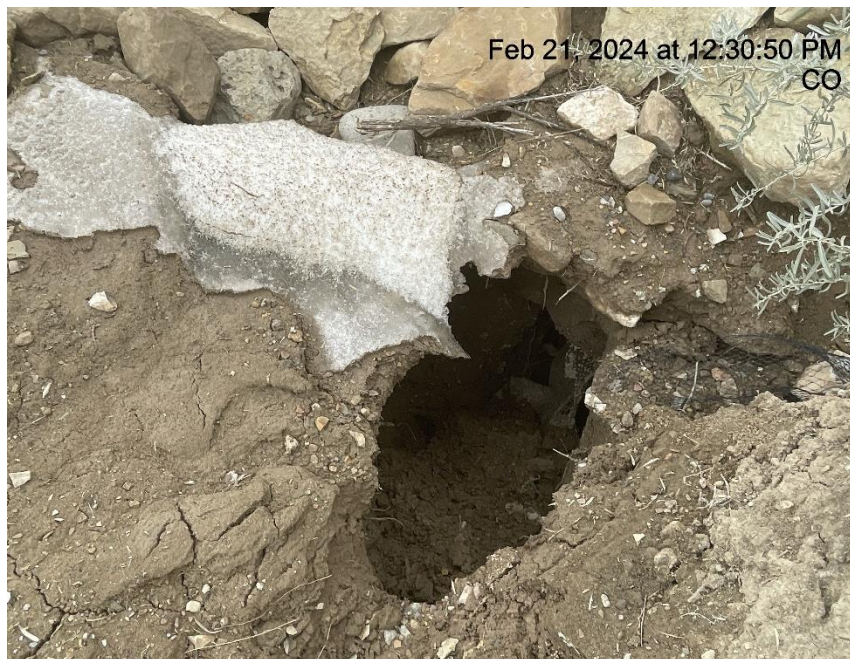
Photo # 7110 Sediment trap needs maintenance
