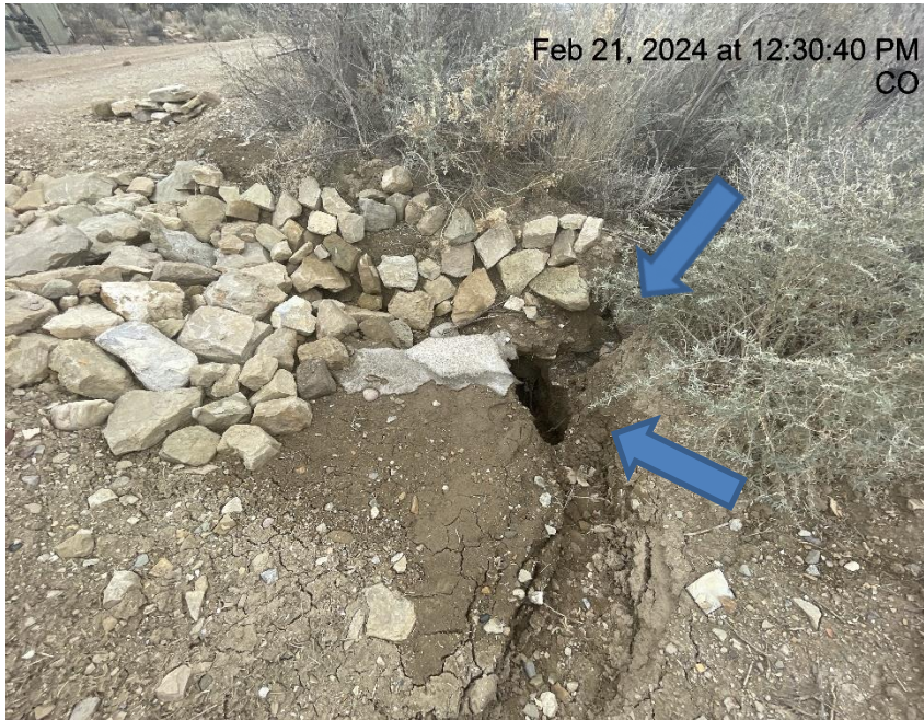
Photo # 7108 Sediment trap needs maintenance
