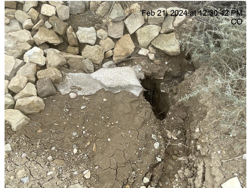
Photo # 7109 Sediment trap needs maintenance
