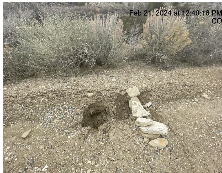
Photo # 7111 Check dam & berm need maintenance
