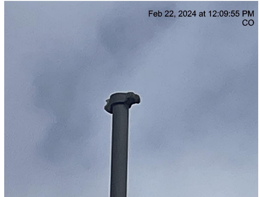
Photo # 7421 Rupture disc vent line lacks cap
