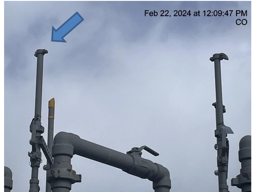
Photo # 7419 Rupture disc vent line lacks cap
