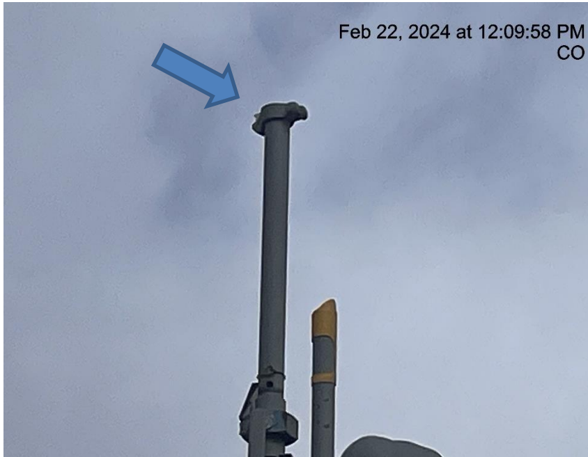
Photo # 7420 Rupture disc vent line lacks cap
