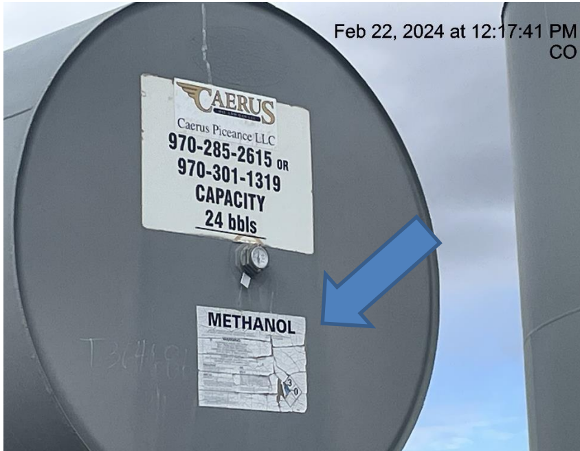
Photo # 7422 Methanol chemical label weathered, cracking & some info becoming illegible.
