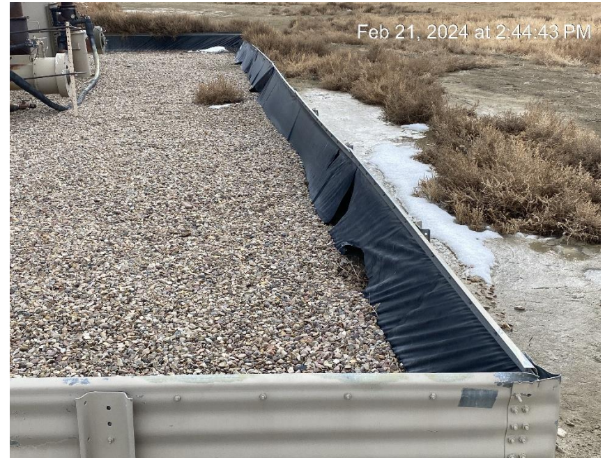
Liner in state of disrepair
