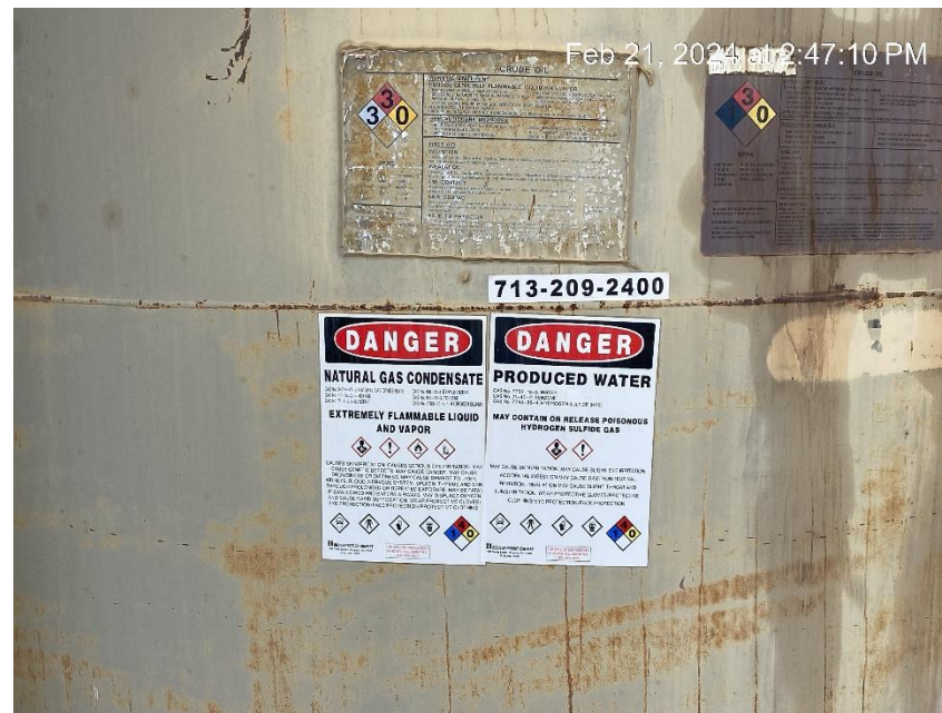
Conflicting and missing required information tank labels
