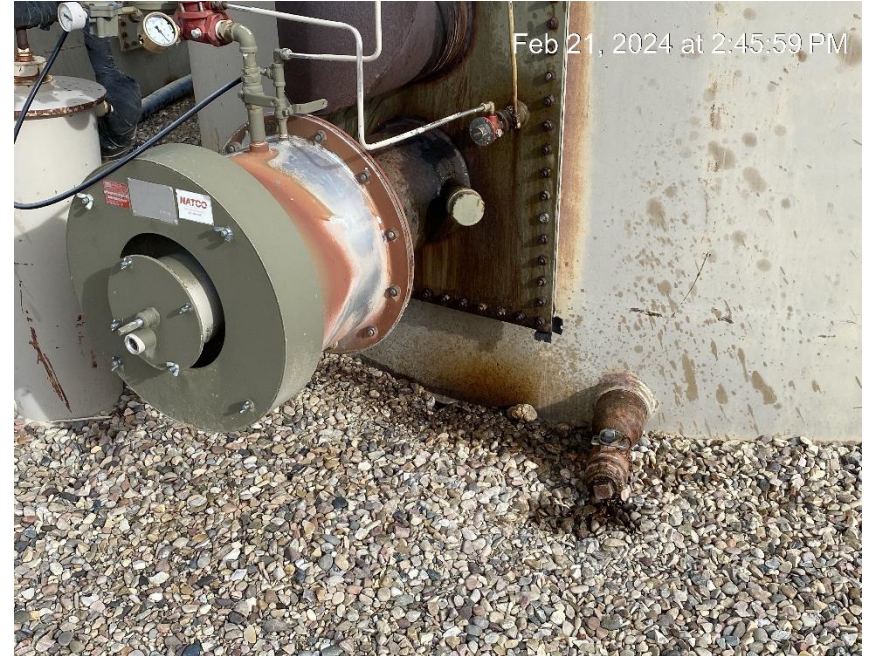
Oily waste and soil staining
