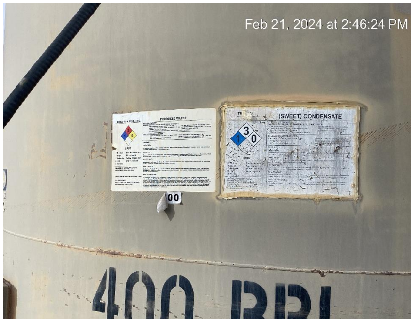
Conflicting and missing required information tank labels
