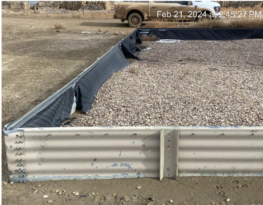
Liner in state of disrepair
