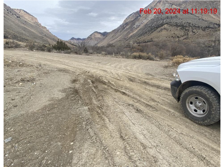
Insufficient Vehicle Tracking BMPs at Location Entrance/Exit – Photo #09404
