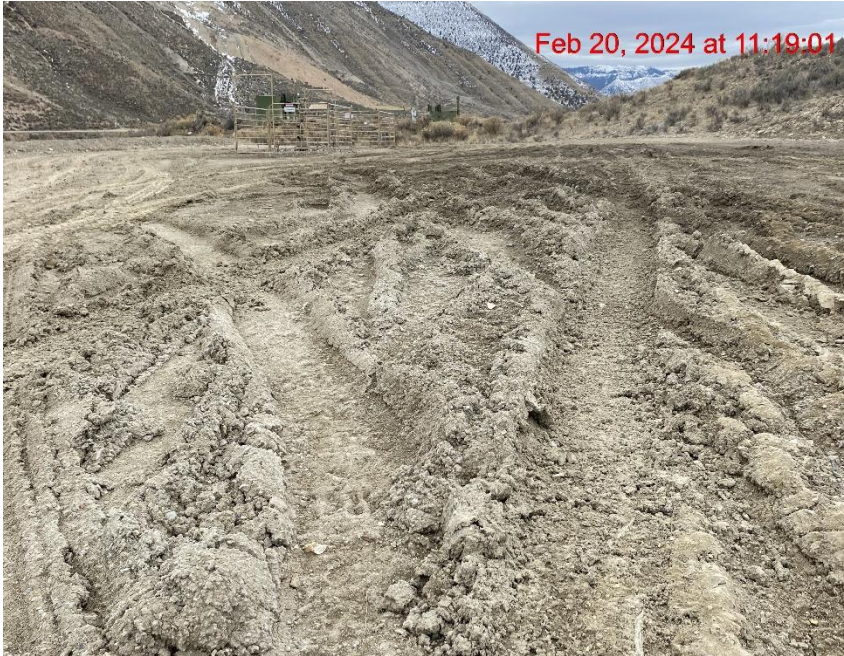
Lack of Stabilization – Photo #09403
