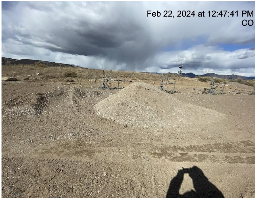
Photo # 7468 Stockpiled soils with no BMP's
