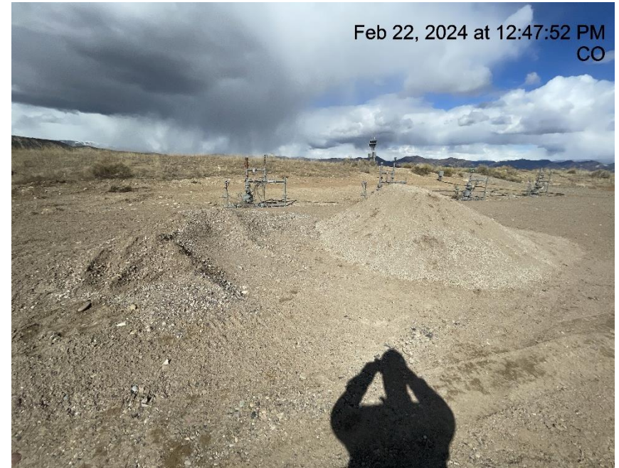
Photo # 7469 Stockpiled soils with no BMP's
