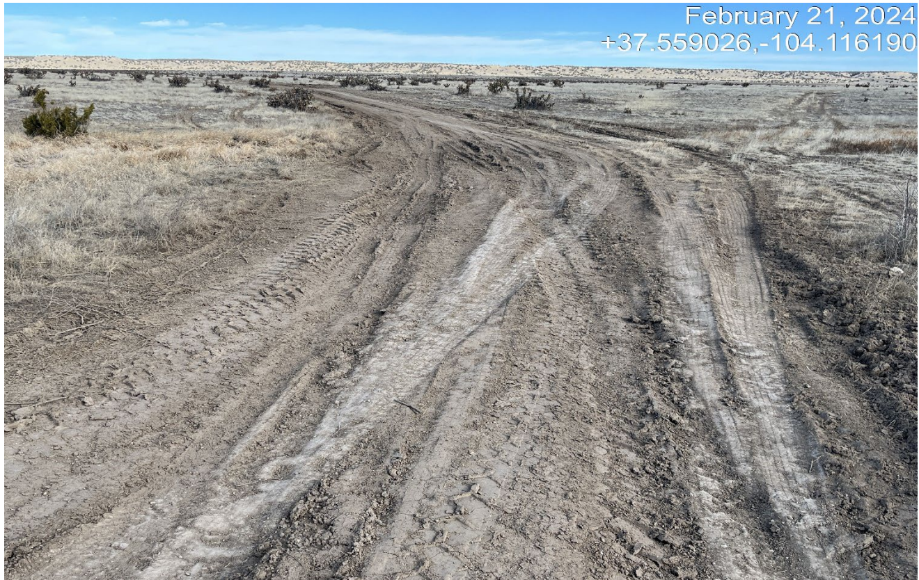
Photo 2. Facing north along the road. There is vehicle rutting that needs to be repaired and the road needs to be maintained to prevent widening and unnecessary disturbance.
