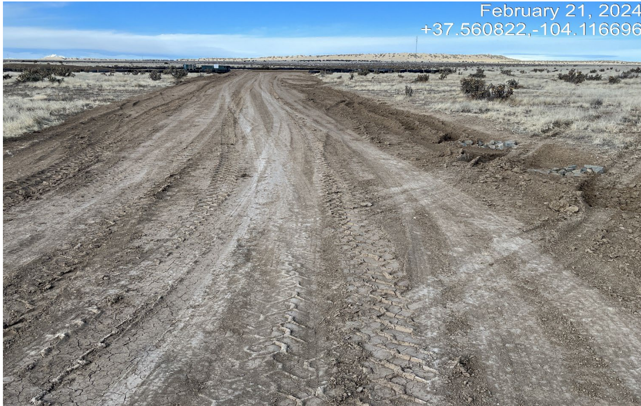
Photo 3. Facing west toward the access road. The side of the road needs to be seeded and stabilized and the road needs to be crowned and graveled if the well is developed. Disturbance needs to be better minimized.
