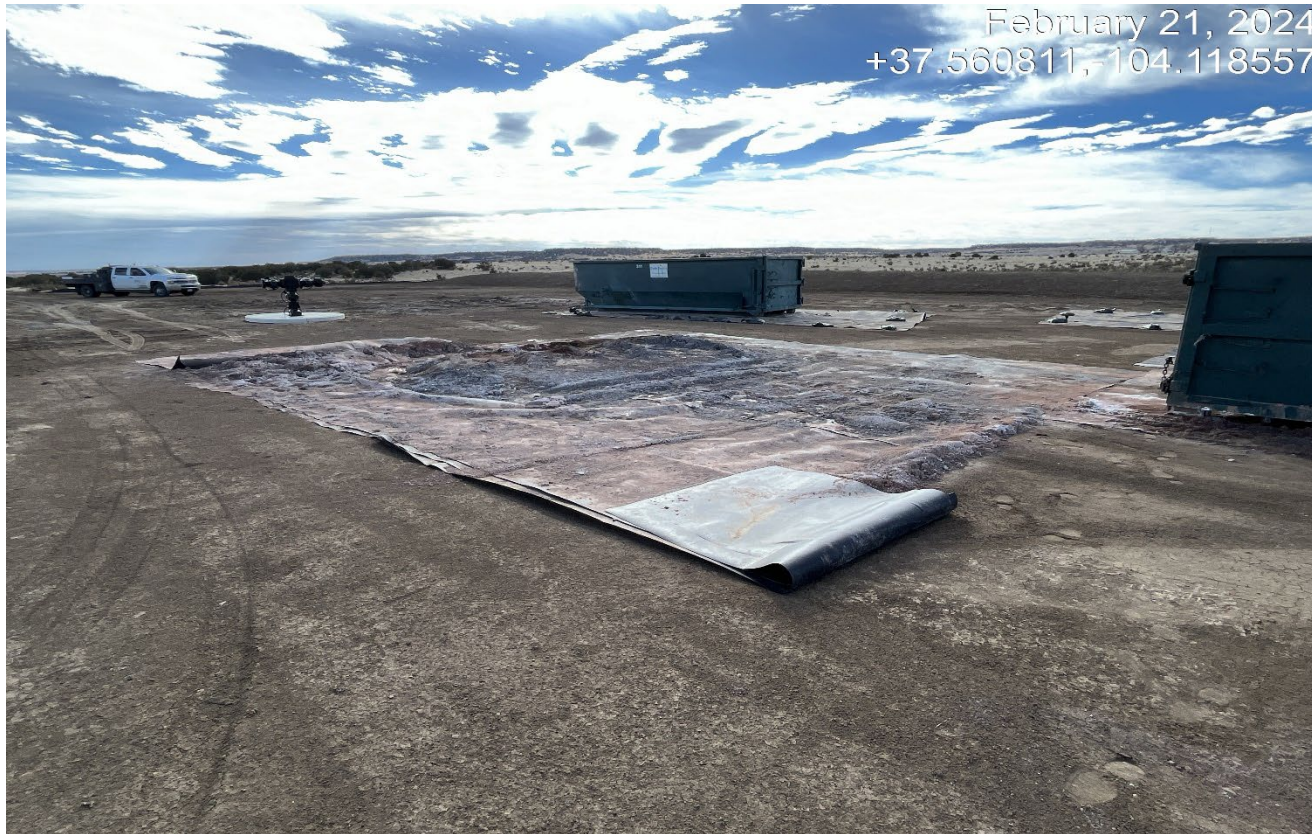
Photo 6. The drill cuttings are not properly stored with containment and have spread off the liner.
