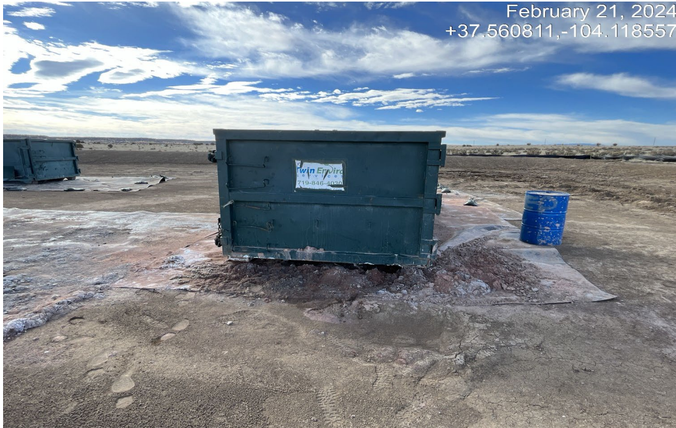
Photo 7. The containers are filled with drill cuttings and appear to be leaking out from the back gate. The drill cuttings are not properly stored with containment and have spread off the liner.
