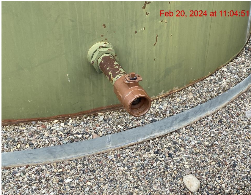
Open-Ended Line on Tank – Photo #09382
