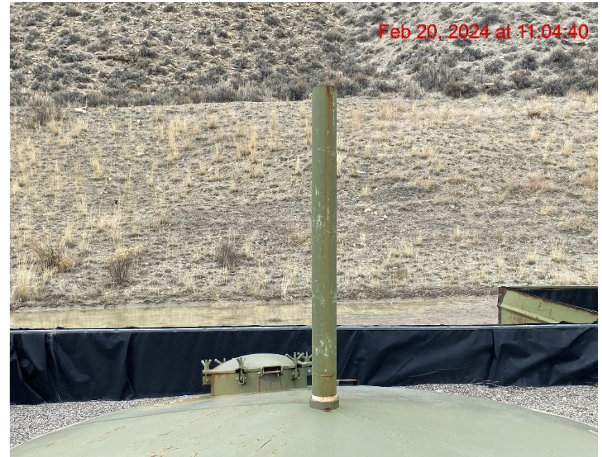
Open-ended/Unprotected Tank Vent – Photo #09381
