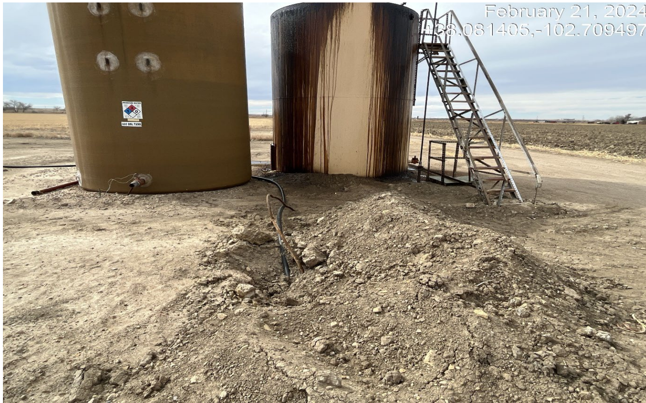
Photo 4. Facing west toward the tank battery which had been significantly remodified and requires secondary containment per Rule 603.o.
