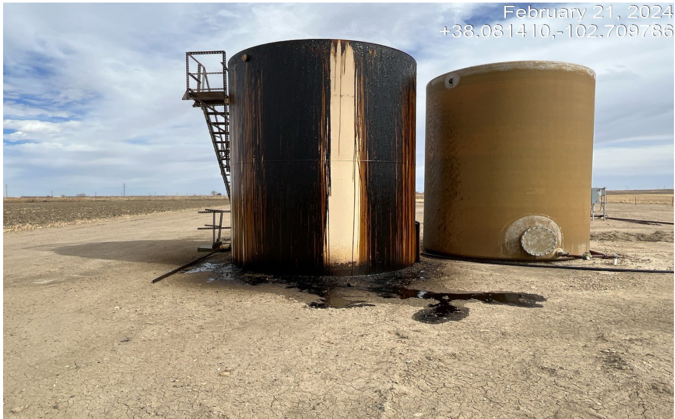
Photo 2. There tank was leak out crude oil at the time of inspection. Operator was immediately notified by phone call. There is no secondary containment to contain the spill as was required by previous inspection.
