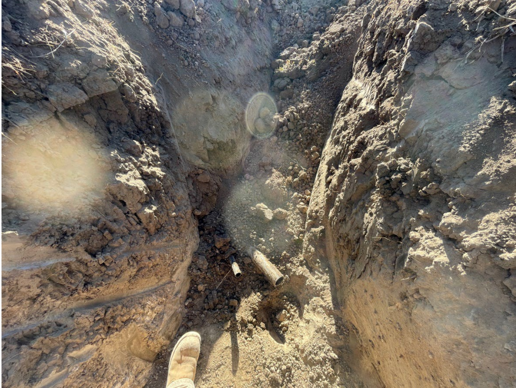
FL4)- Flowline sample location at wellhead (FLN1) Staining and odor observed
