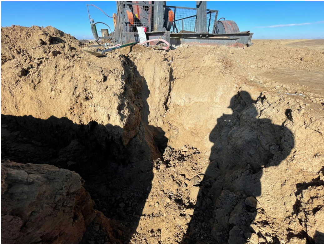
FL4)- Flowline sample location at wellhead (FLN1) Staining and odor observed
