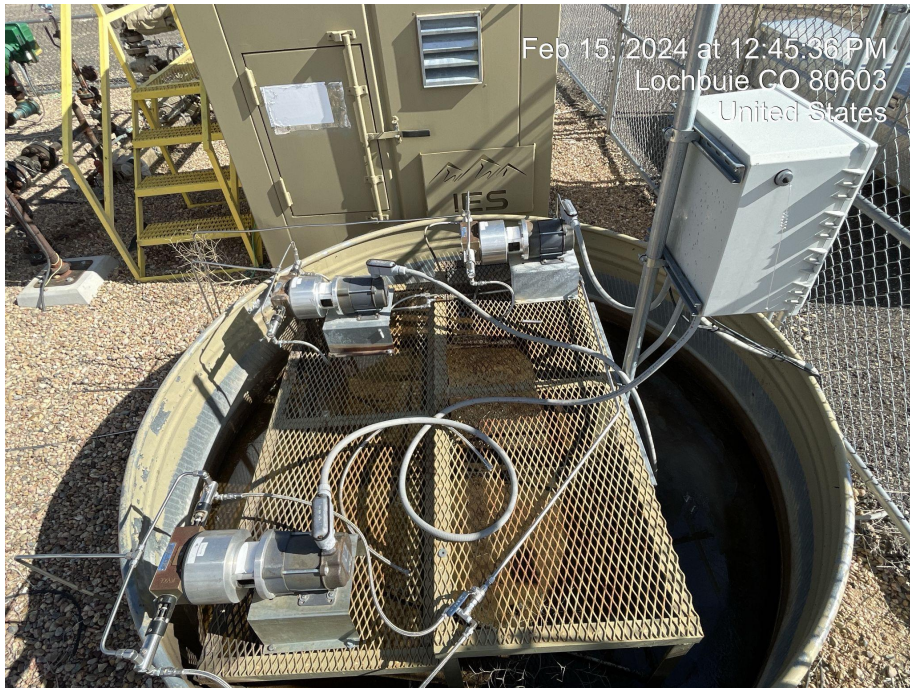
Photo 5. Photo taken of secondary containment on well pad missing wildlife protection. Photo taken facing east.
