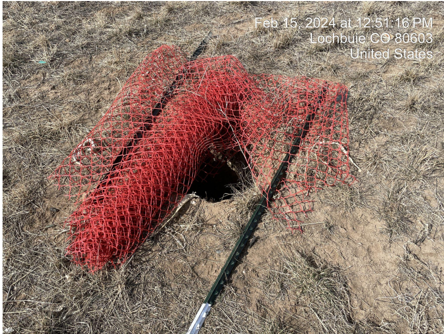
Photo 9. Photo taken of potholes lacking proper fencing on perimeter of location. Photo taken facing west.
