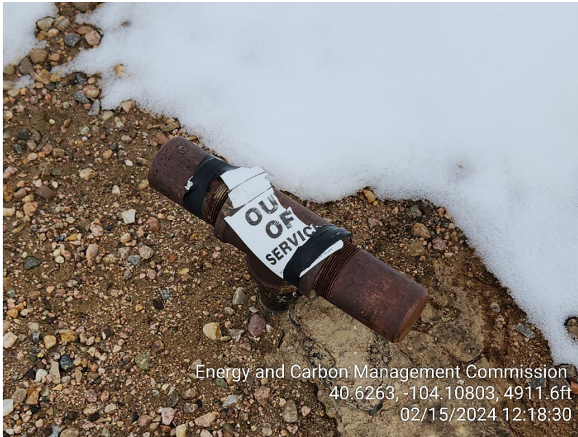
Photo 3 – Tag has weathered
