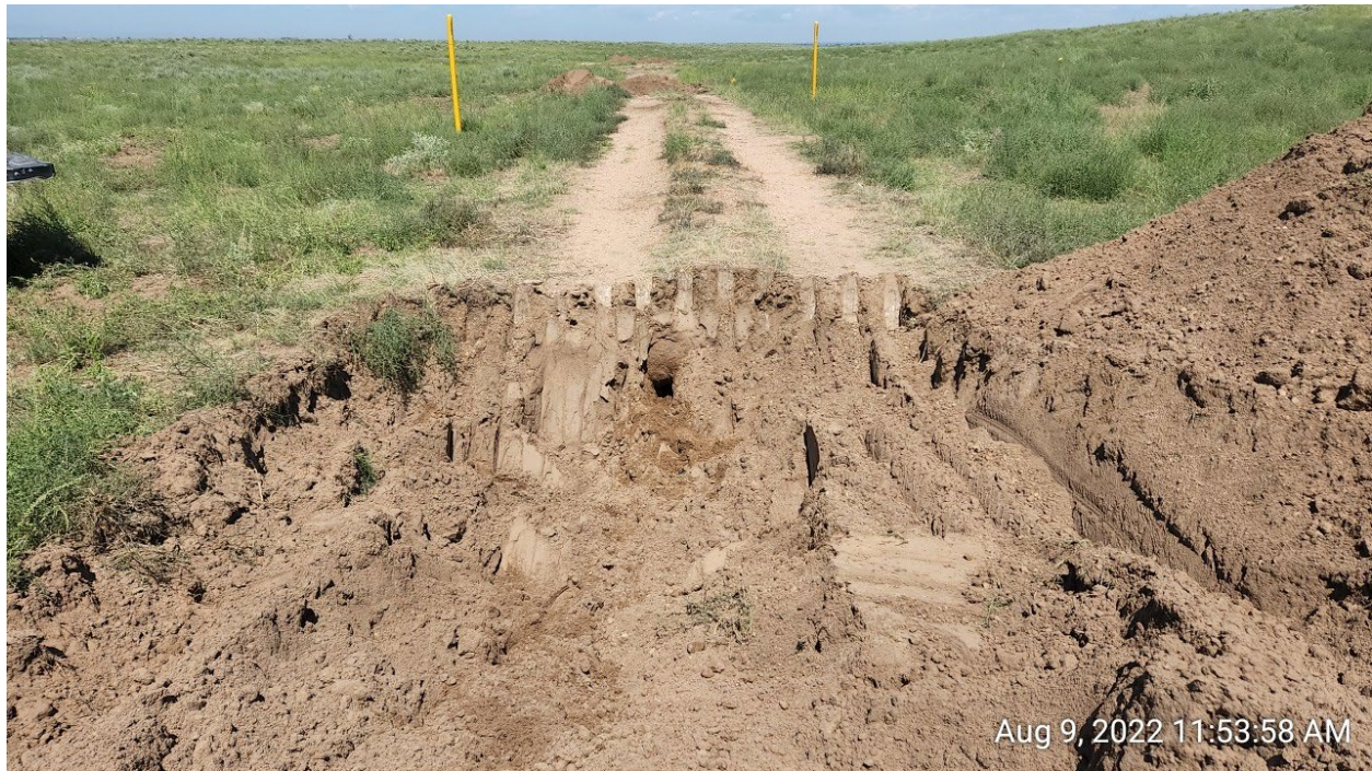
#1C – State 36-9i4 Flowline – 9FL03@3.0' – Odor Present – PID 284.7ppm – Sample Submitted for Lab Analysis
