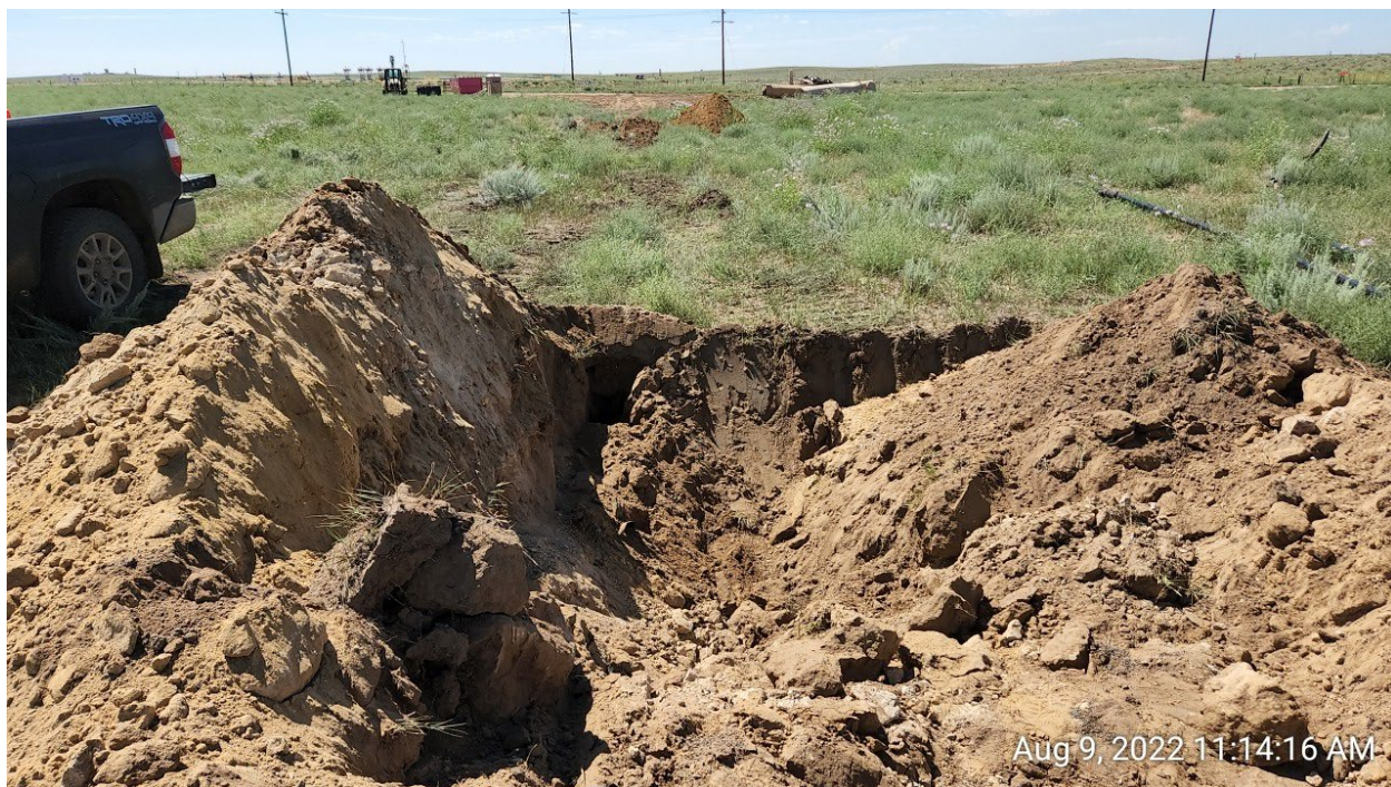
#1I – State 36-9i4 Flowline – 9FL09@3.0' – Odor Present – PID 2628ppm – Sample Submitted for Lab Analysis
