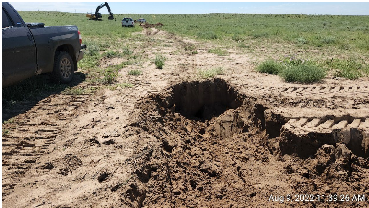
#1A – State 36-9i4 Flowline – 9FL01@3.0' – No Impacts Noted – PID 274.0ppm – Sample Submitted for Lab Analysis
