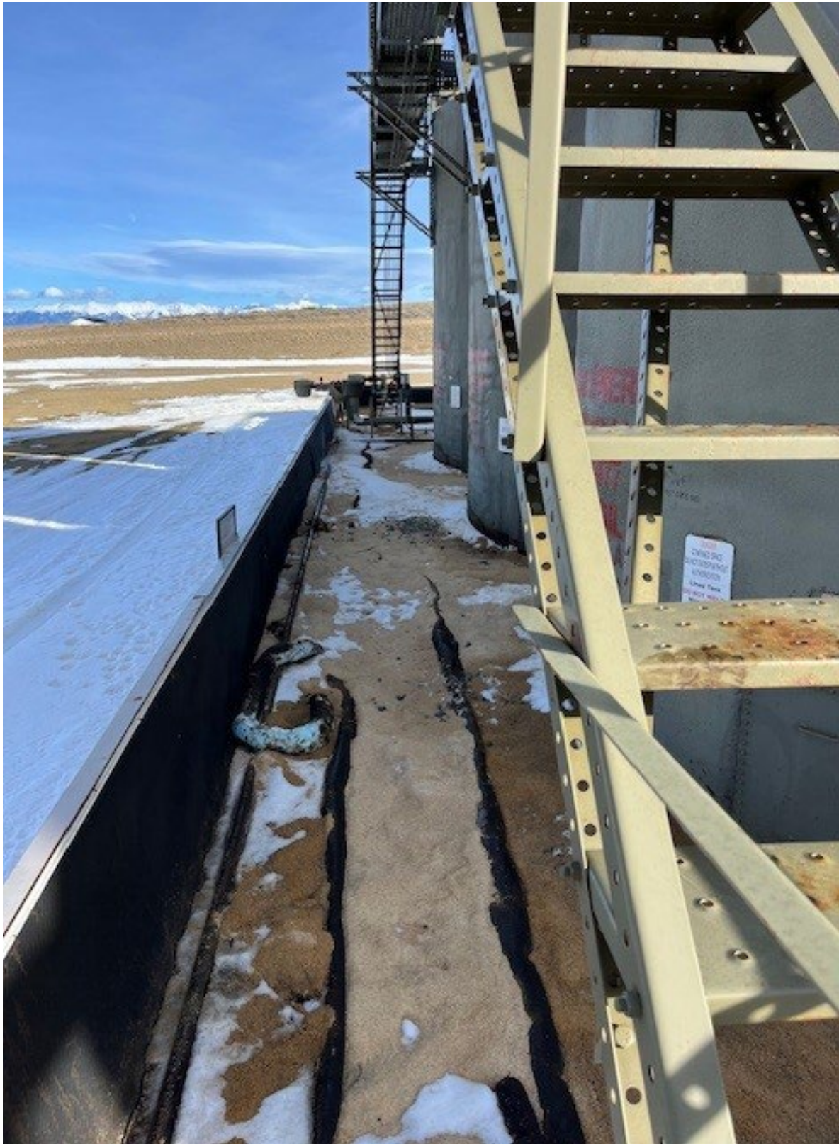
PHOTO NO 2: NORTHERN EDGE OF CONTAINMENT LOOKING EAST
