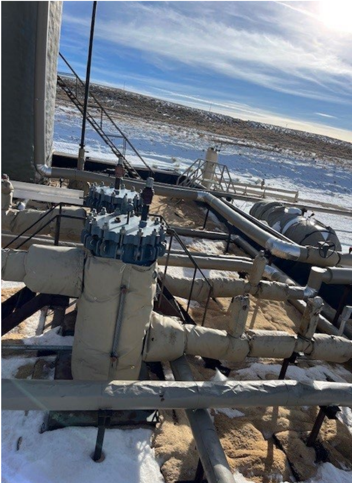
PHOTO NO 7: SPILL AREA LOOKING SOUTH FROM NW CORNER OF CONTAINMENT
