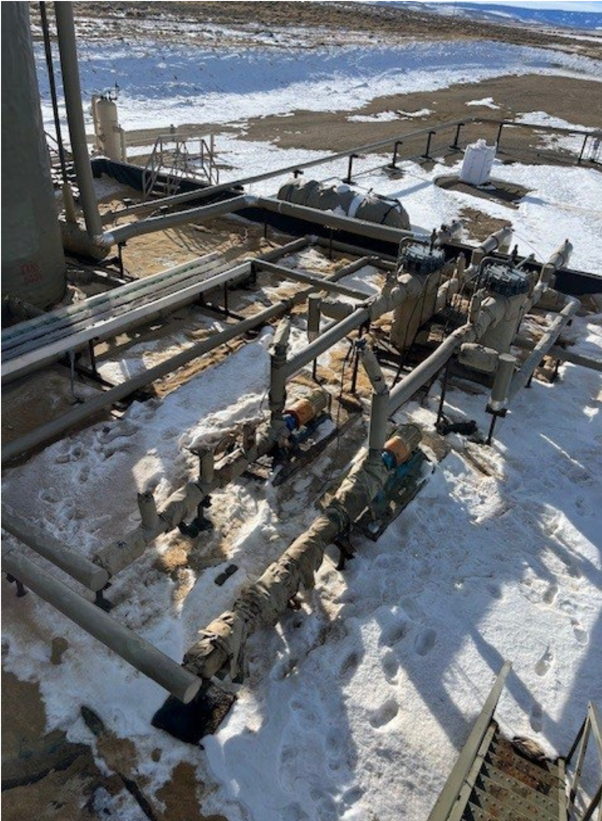
PHOTO NO 1: LOOKING INTO NW CORNER OF CONTAINMENT FROM POINT OF NW TANK
