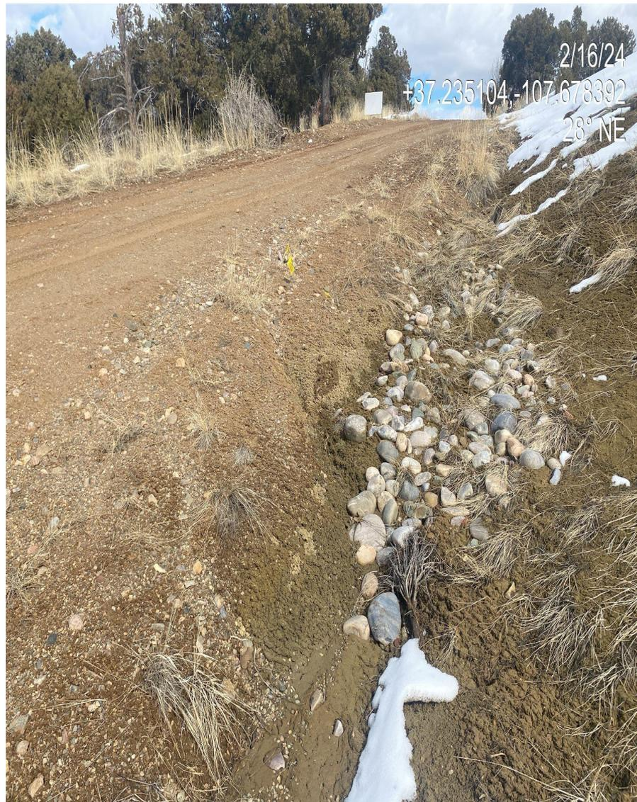
**Photo 3.** View of rill erosion forming in the southern interim reclamation and along the eastern edge of the access road.
