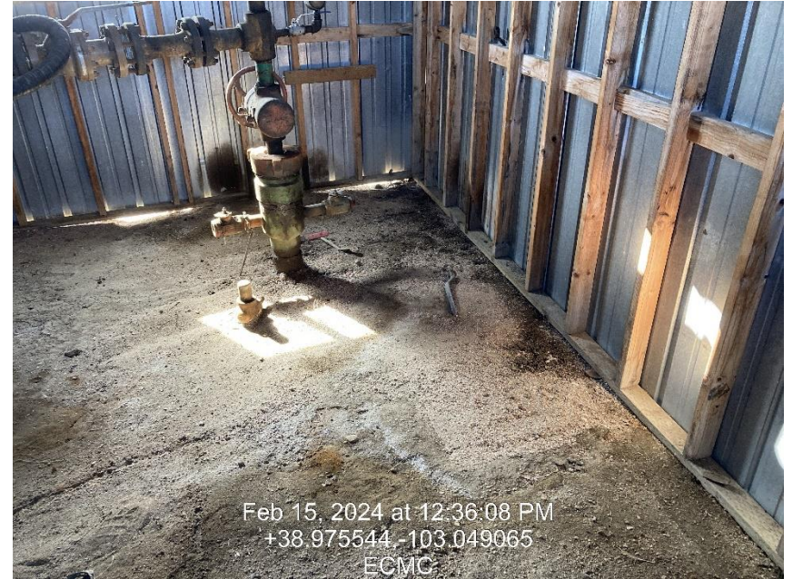
Photo 4 – – Impacted soil observed inside wellhead building
