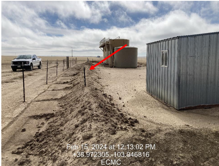
Photo 5 – Containment Berm on West side of Tank Battery
