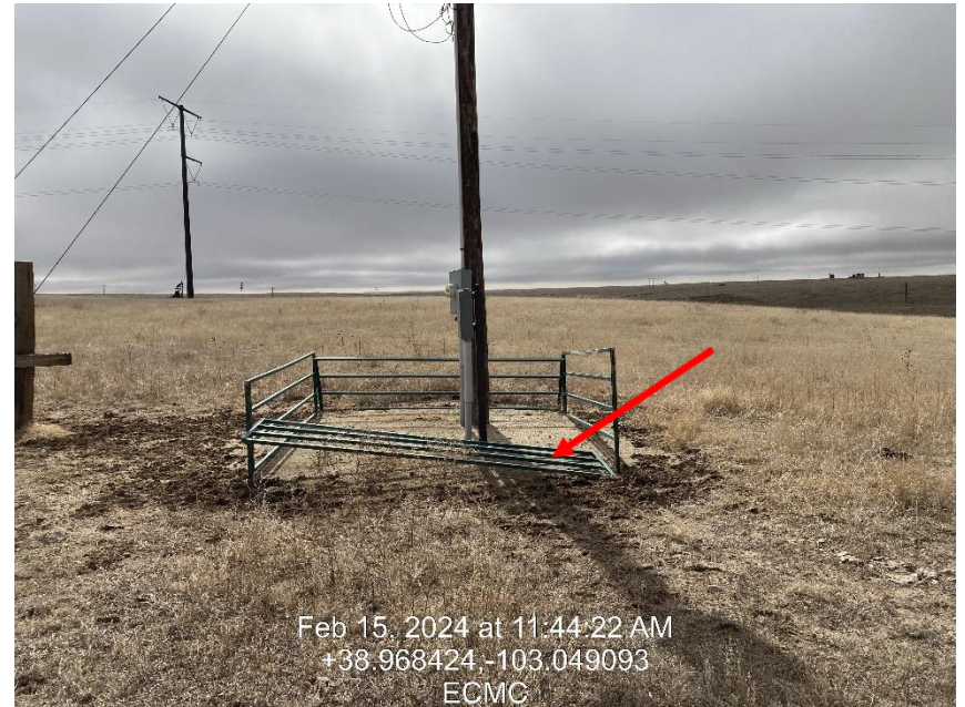
Photo 4 – Guarding not maintained, Electrical drop
