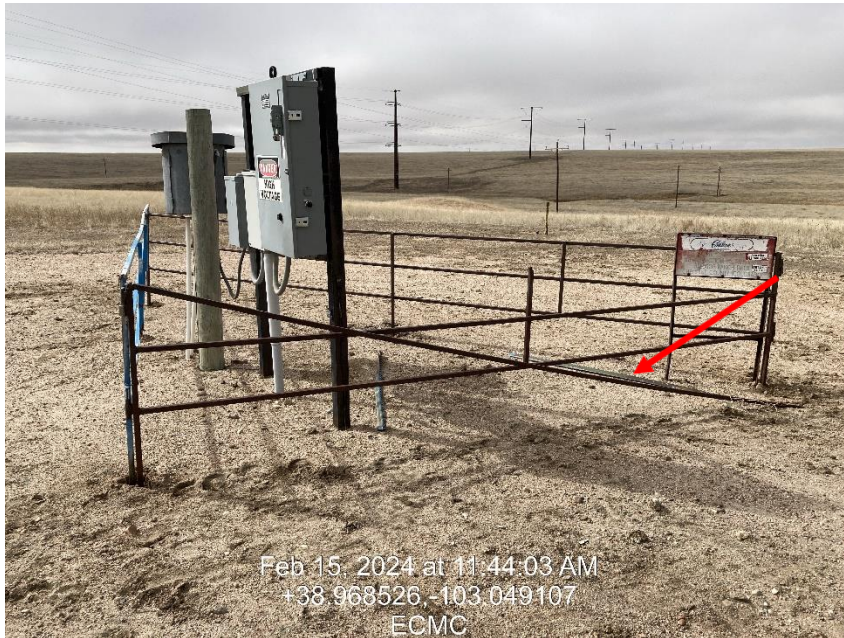
Photo 3 – Machine Guarding not maintained. Electrical Panel and Rectifier
