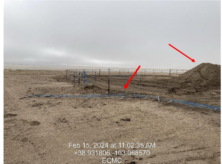
Photo 10 – Soil pile, Fencing/Guarding not maintained
