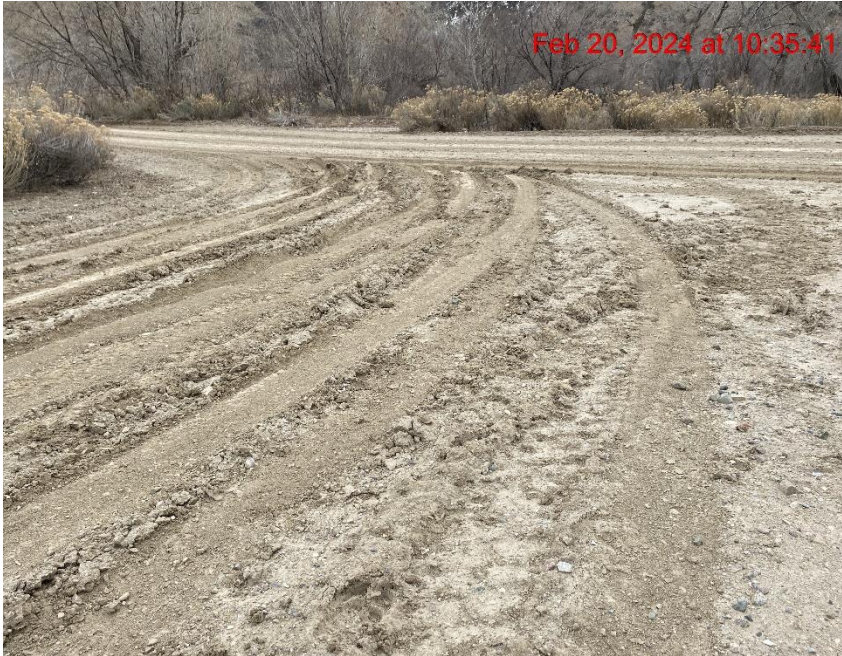
Insufficient Vehicle Tracking BMPs at Location Entrance/Exit – Photo #09344
