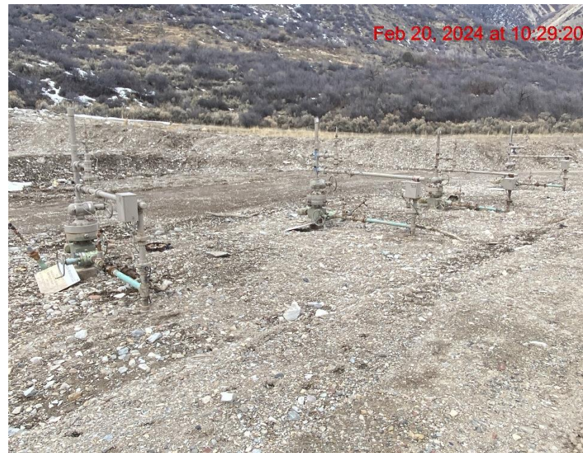
Wellhead/Signs Not Posted or Visible – Photo #09335
