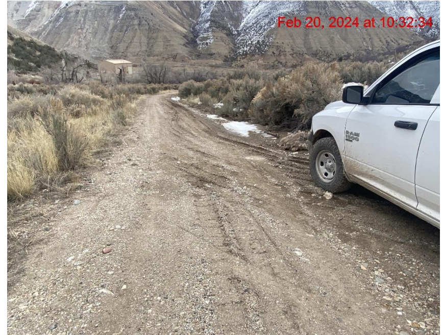
Insufficient Vehicle Tracking BMPs at Location Entrance/Exit – Photo #09342
