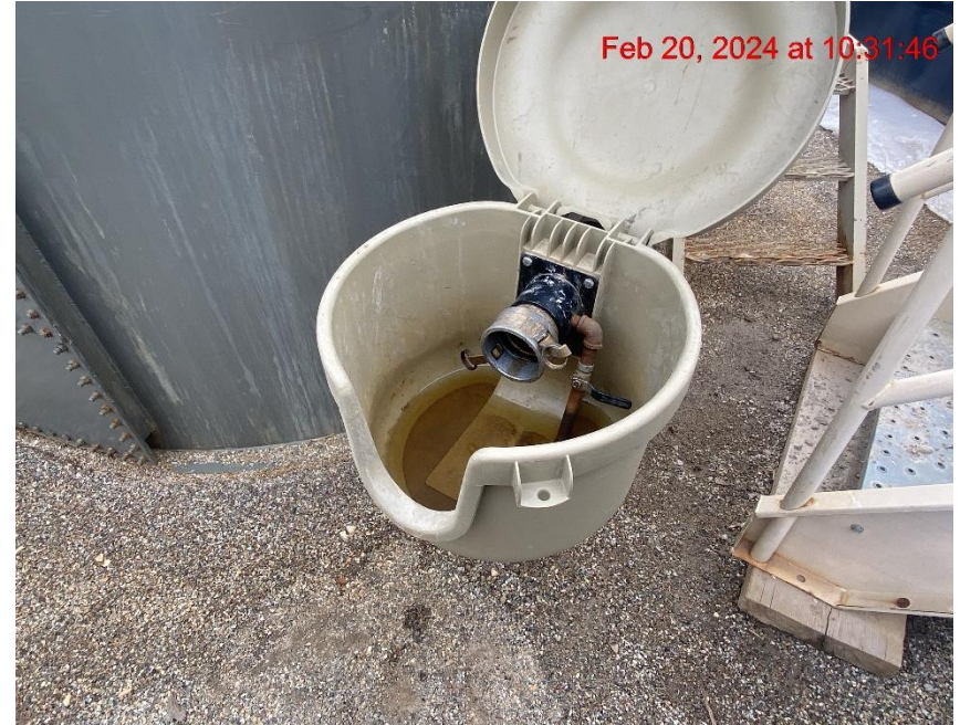
Open-Ended Load Line – Photo #09340
